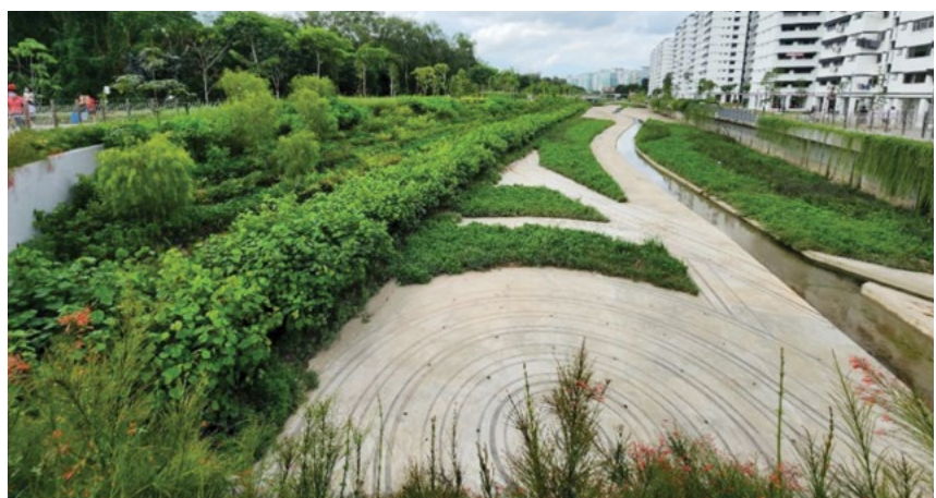
Figure 8: Bio-engineered, sloping river bank after completion, with vegetation fully grown.
