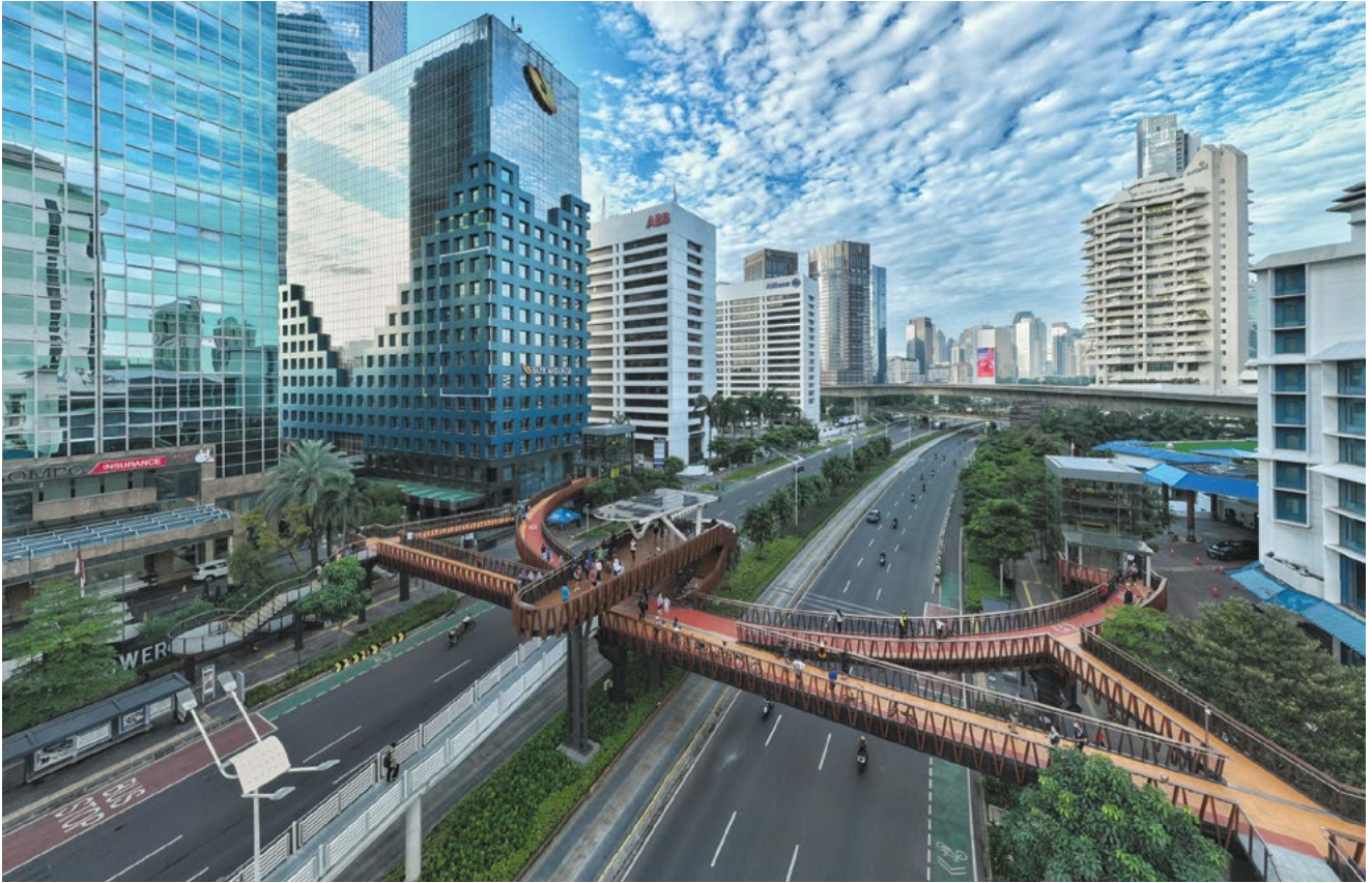
The Pinisi Crossing Bridge, with high-rise buildings in the background.
