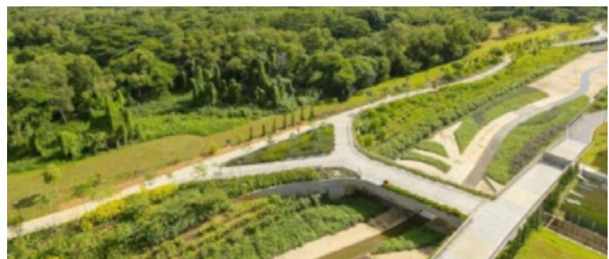
Figure 10: Aerial view of the completed ABC water project at Sungei Tampines, highlighting the innovative implementation of the geogrid-reinforced, soil bio-engineered slope with vegetation, as a natural river bank.
