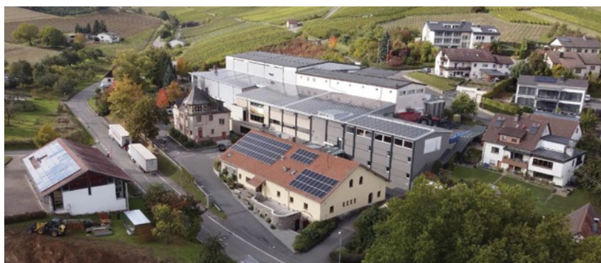
Systemair upgraded the ventilation system at Beckstein winegrowers' cooperative, founded 1894 in Germany, by replacing an old axial fan with modern MUB fans featuring EC technology.
