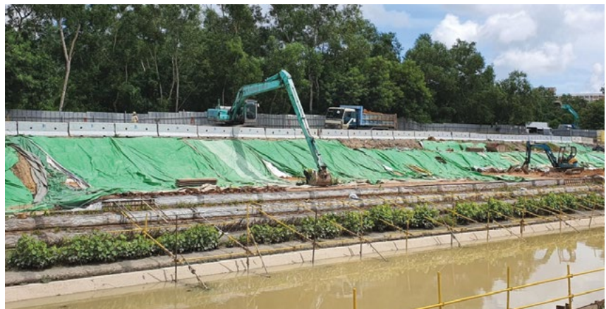
Figure 7: View of the bio-engineered, sloping river bank during construction.
