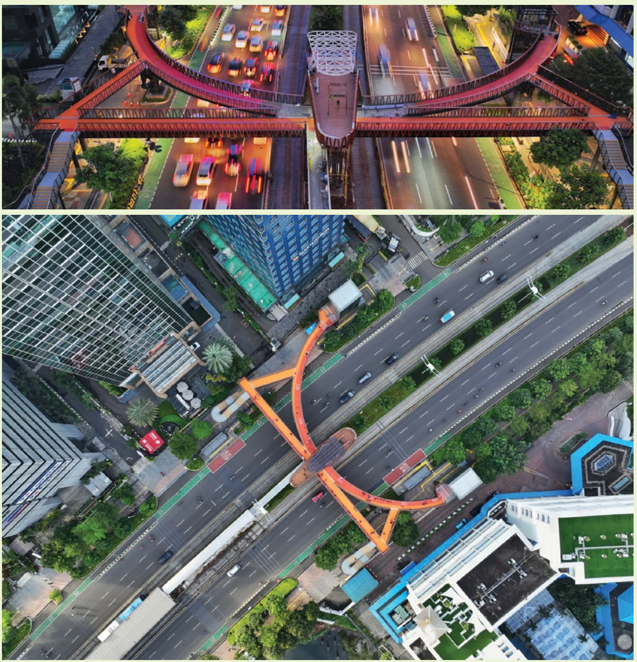
Aerial views of the 'K-shaped bridge.
