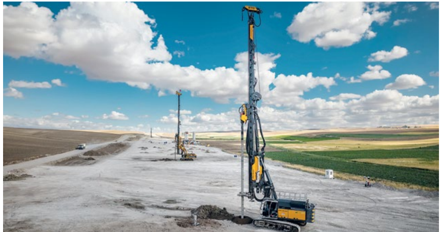
In the resource-efficient single column mixing method, the existing in-situ ground is mixed with a binding agent. Single columns are produced after hardening.
