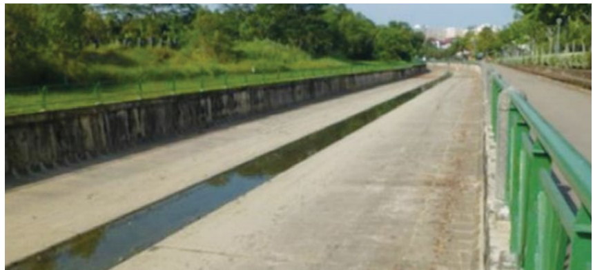
Figure 1: Conventional concrete-lined drain for storm water management.
