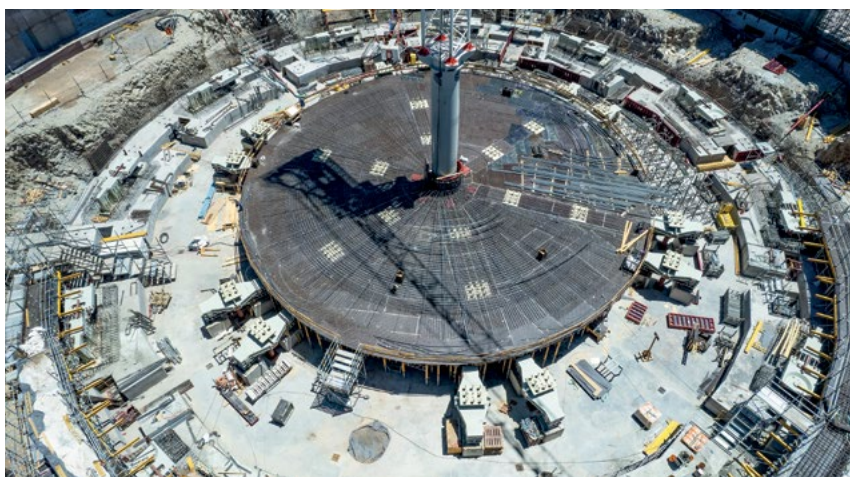
A bird's-eye view of the base of the ELT, which was formed with the MULTIFLEX Girder Slab Formwork.
