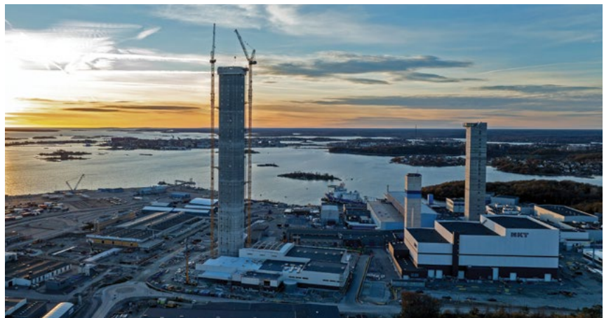
Thanks to an innovative crane solution, the tower was erected in just 90 days.
