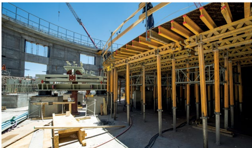
MULTIFLEX Girder Slab Formwork for fast and flexible covering of the base of the ELT.
