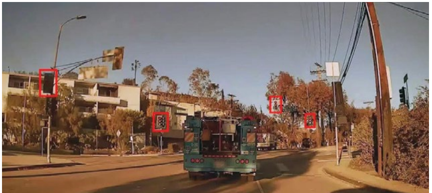
Malfunctioning streetlights are detected by Bentley's Blynscsy technology in crowdsourced dash cameras in the Los Angeles area after wildfires caused major damage to critical safety infrastructure. Image: Bentley Systems.
