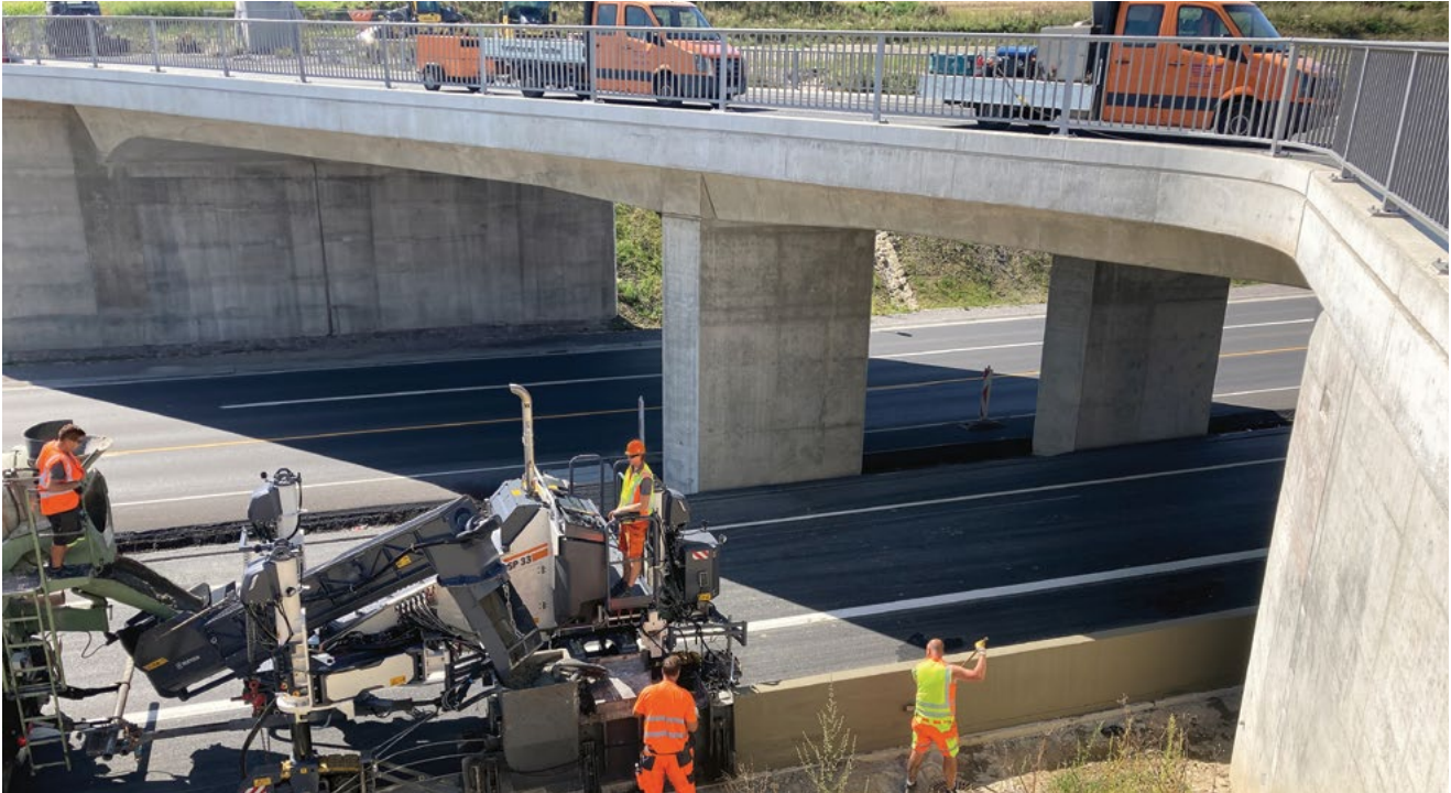
The Wirtgen SP 33 can pave a wide range of different monolithic concrete profiles, e.g. kerbs, kerb gutter profiles, rectangular profiles, concrete barriers up to 1.3 m in height or sewers and drainage channel profiles.
