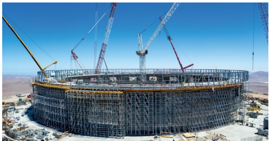
By combining the ST 100 Stacking Towers with components from the PERI UP Scaffolding Kit, access to the platform above could be created.
