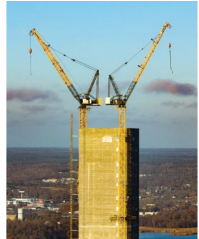
The Liebherr 542 HC-L and 258 HC-L cranes.
