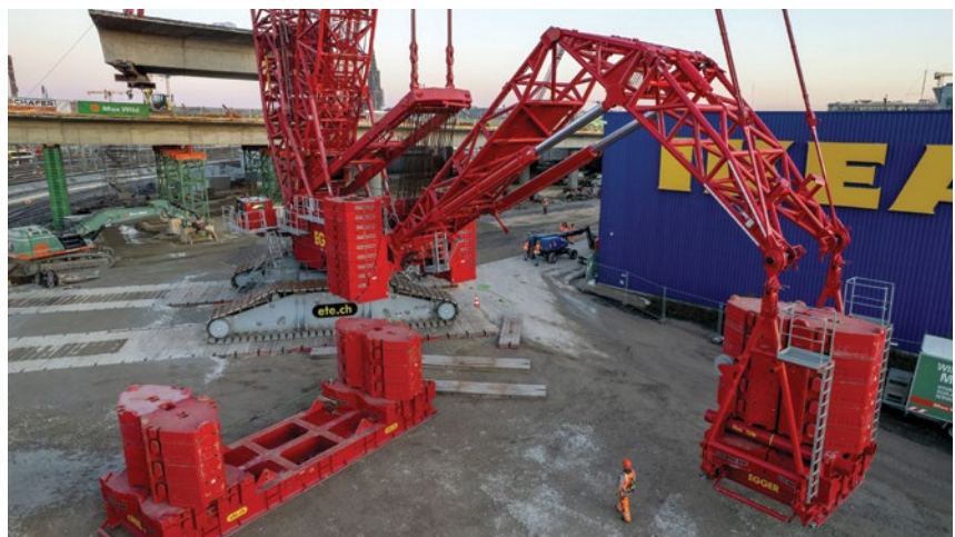
The hydraulically adjustable V-Frame folding frame and the divisible VarioTray derrick ballast were valuable features during the operation.
