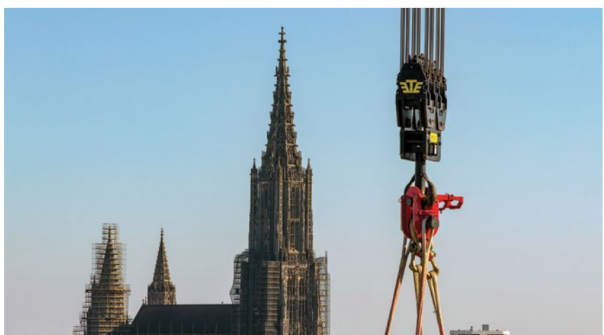
A balancing mechanism on the hook block of the crawler crane ensured that the load was evenly distributed across all four Dyneema ropes.
