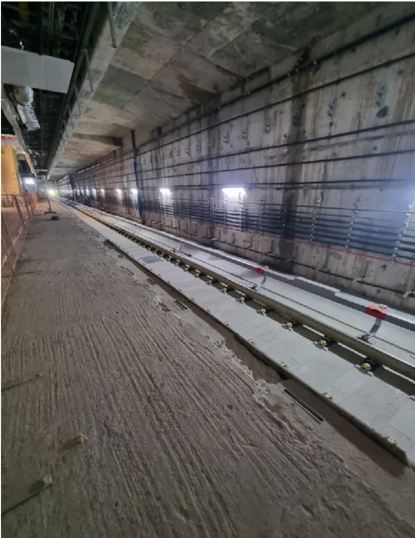
Preparation works for installation of platform screen doors on the Downtown Line MRT Extension.
