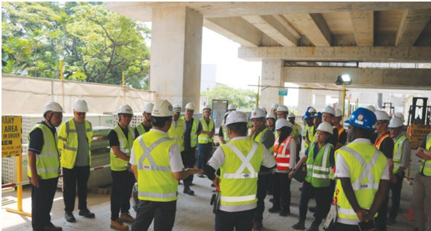
Site visit to the JW5 Station.
