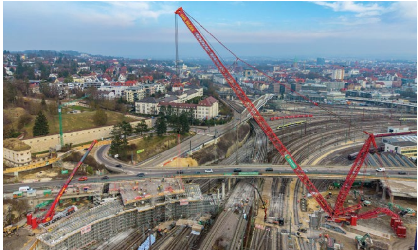
In order to reach the more distant segments, the main boom of the Liebherr LR 11000 was extended from 84 m to 128 m. On the left of the picture is the LTM 1650-8.1 mobile crane.
