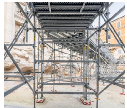
The scaffolding supports were placed on rubber pads and wooden boards to protect the vulnerable surface of the Trevi Fountain. Image: PERI SE.
