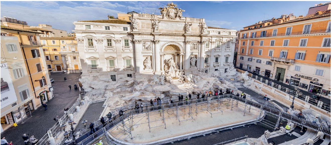
The temporary scaffolding solution had a load-bearing capacity of 500 kg/m 2 , thus offering maximum stability and safety, even with high visitor numbers. Image: PERI SE.
