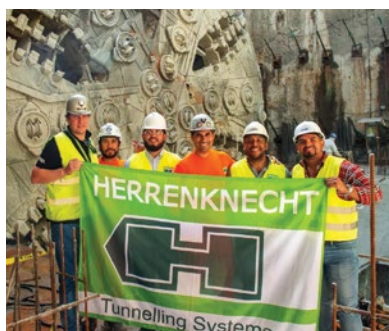
Members of the Herrenknecht team, after the successful intermediate breakthrough to the future Balboa metro station.
