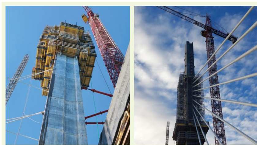
SKE100 plus and SKE50 plus climbing systems enabled safe and efficient construction of the 102 m pylon.
