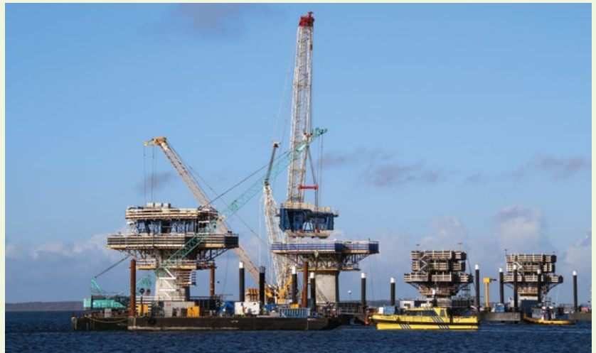
The new Storstrøm Bridge, Denmark's third longest bridge, forms part of a continuous connection between Scandinavia and Central Europe.
