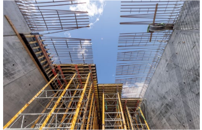
MULTIPROP Shoring Towers are used as a supporting structure for concreting the slab, ensuring that this work can be carried out safely.
