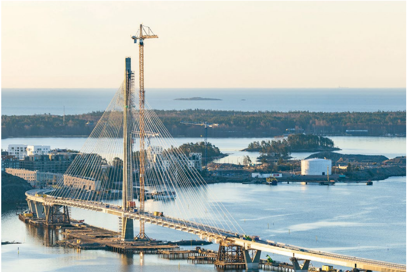
The Kruunuvuori Bridge, centrepiece of the ambitious Kruunusillat (Crown Bridges) project, is one of the most technically demanding infrastructure projects currently under construction in Northern Europe.
