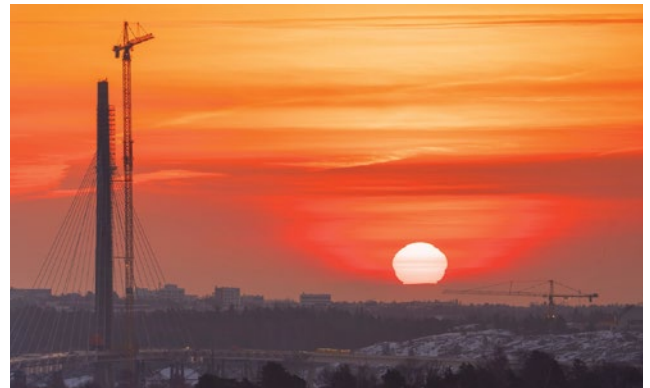
At the heights involved, with the crane mast tied into a pylon structure that itself rises 135 m, both the static and dynamic wind forces acting on the crane assembly had to be carefully assessed.
