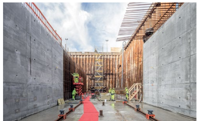
The tunnel is being constructed using the cut-and-cover method, with the bottom plates, walls and slabs being concreted in succession across 54 sections.
