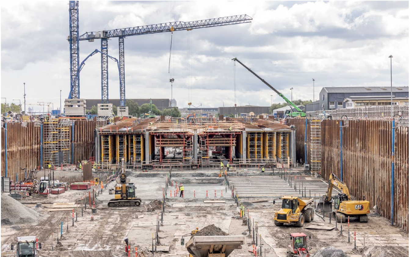
The 1.4 km long Nordhavn Tunnel in Copenhagen is being constructed as a twin-tube tunnel, with separate directions of travel.
