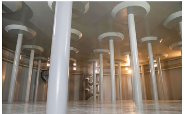
Interior of Tengah Service Reservoir Tank 1. Image: PUB.
