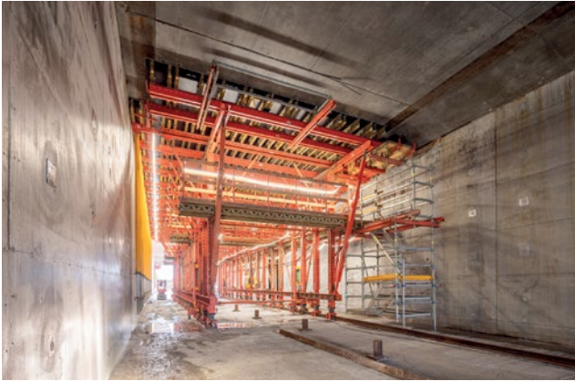
Eight VTC Tunnel Formwork Carriages enable precise and repeatable concreting cycles, ensuring steady construction progress on the Nordhavn Tunnel.
