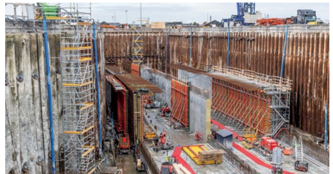
PERI formwork and scaffolding systems are used on the construction site and are tailored to work seamlessly together.
