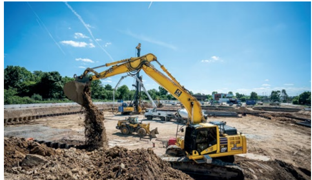
The Semi-GPS 3D excavator grades the subgrade with an accuracy of up to 2 cm. Image: BAUER Group.
