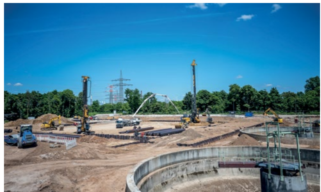
Drone footage documented the progress of construction and the total volume of excavated soil, which amounted to 45,000 m 3 . Image: BAUER Group.
