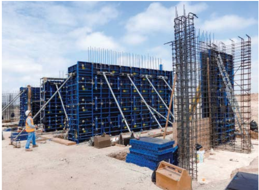
The DokaFit Handset is a lightweight system with integrated ergonomic handles, designed for efficient forming. Image: Doka.
