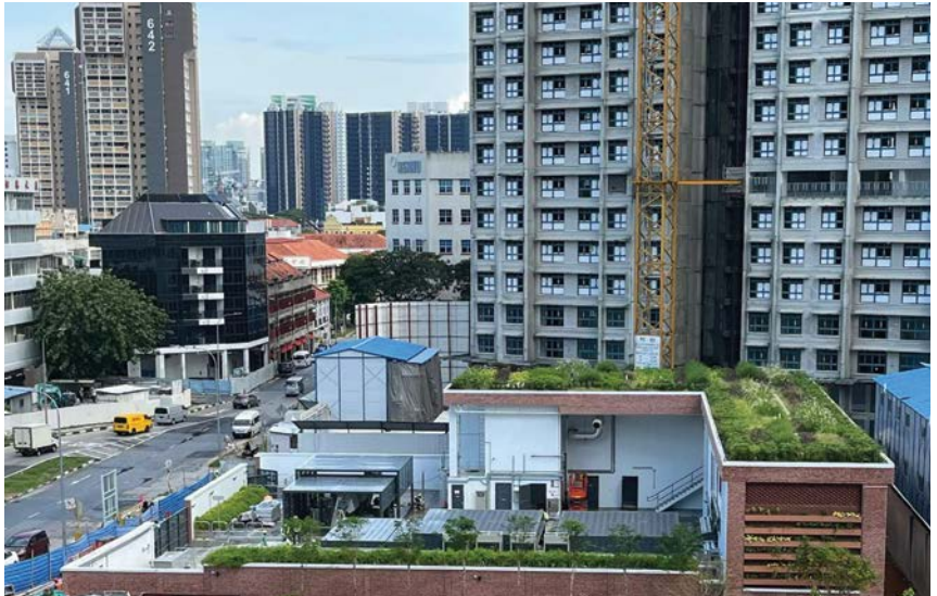
The Syed Alwi Pumping Station forms part of the stormwater management infrastructure in Singapore.
