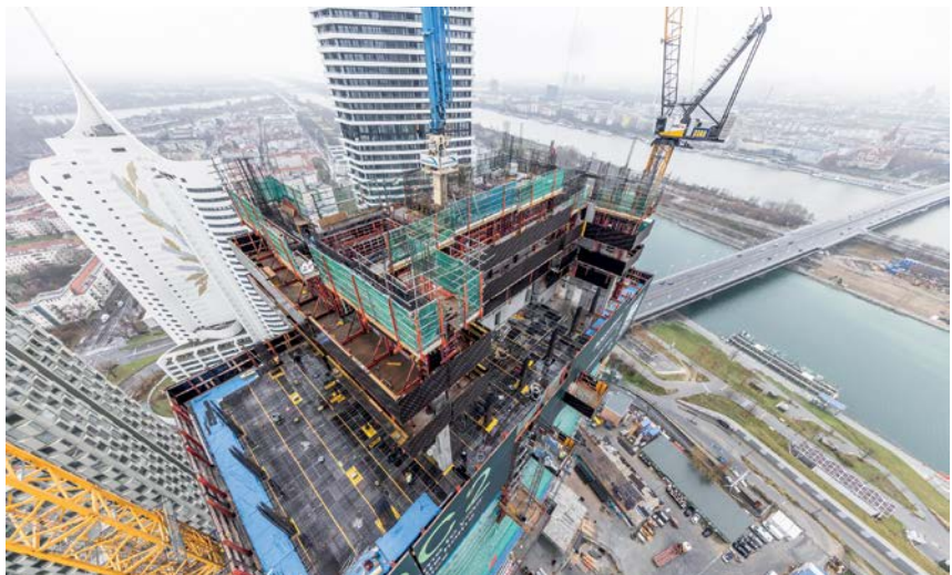
PERI is supporting the construction of DC Tower 2, with formwork and scaffolding solutions. Image: PERI.
