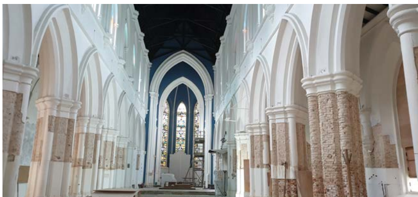
Restoration work was carried out also on the interior walls of the cathedral.
