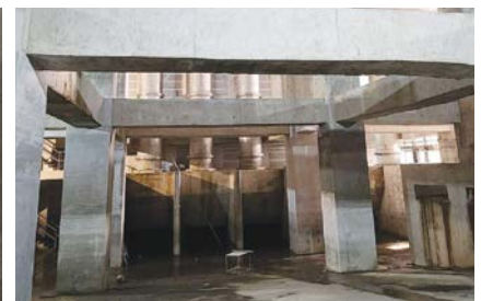
Stormwater passes through raker screens at the inlet (left), that removes debris, before entering the main underground storage tank (right). The tank can hold 9,300 m 3 of stormwater.
