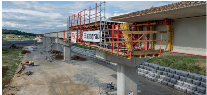
The VARIOKIT VCT Composite Track, a solution for steel composite bridges that won the bauma Innovation Award 2025, is making its début in Croatia.
