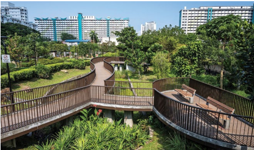
Whampoa Park incorporates Active, Beautiful, Clean Waters (ABC Waters) design features, such as this rain garden that purifies surface runoff before it enters the nearby Sungei Whampoa. Image: HDB.
