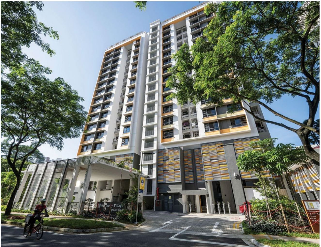
Harmony Village @ Bukit Batok was complex to construct, with residential units, communal facilities for seniors and a hawker centre integrated in a single development. Image: HDB.
