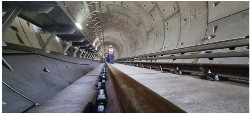
Tunnel inspection works in Shah Alam, Malaysia. Image: Daniel Woods.
