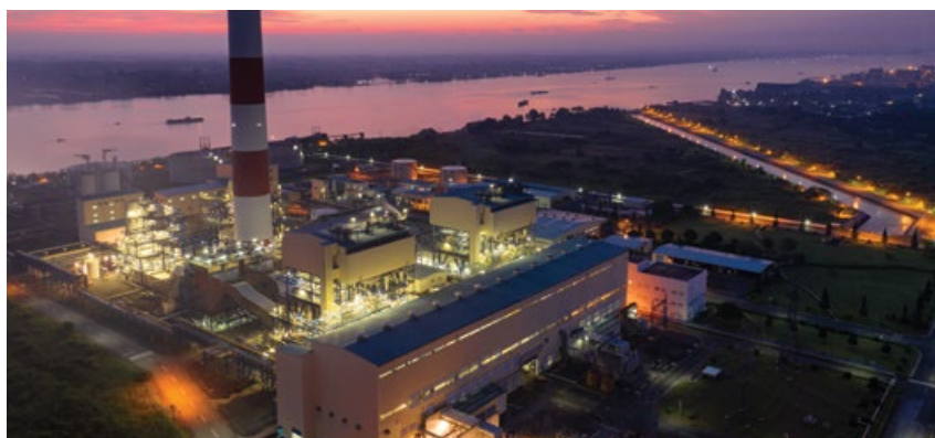
O Mon 1 Thermal Power Plant in Vietnam
