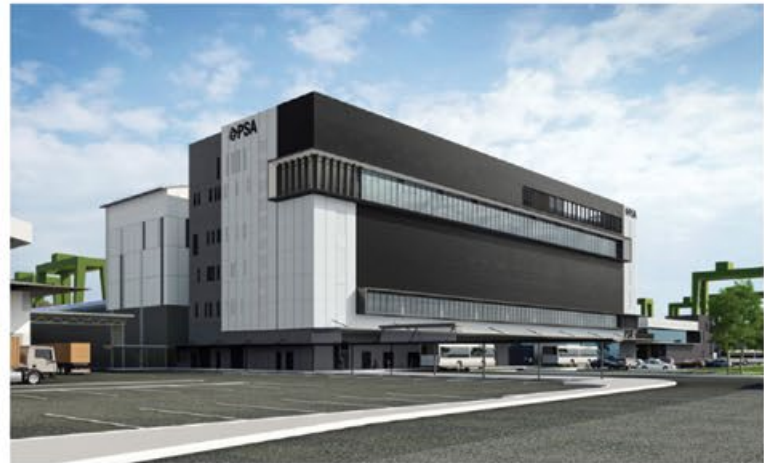
PSA Building – BAPV Façade (Completed 2021)
