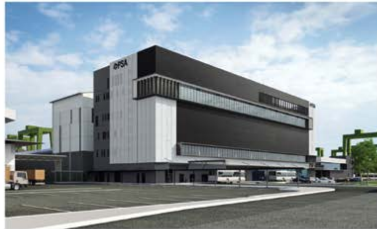
PSA Building – BAPV Façade (Completed 2021)
