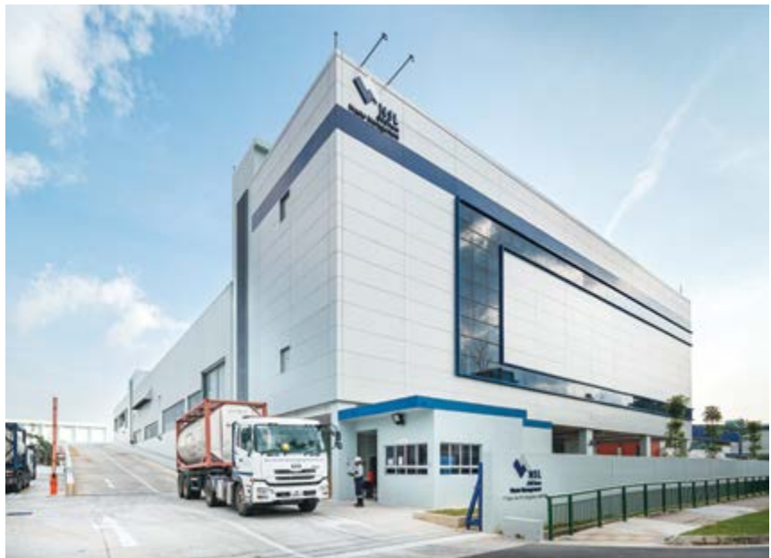
NSL OilChem Waste Management's industrial wastewater treatment hub
