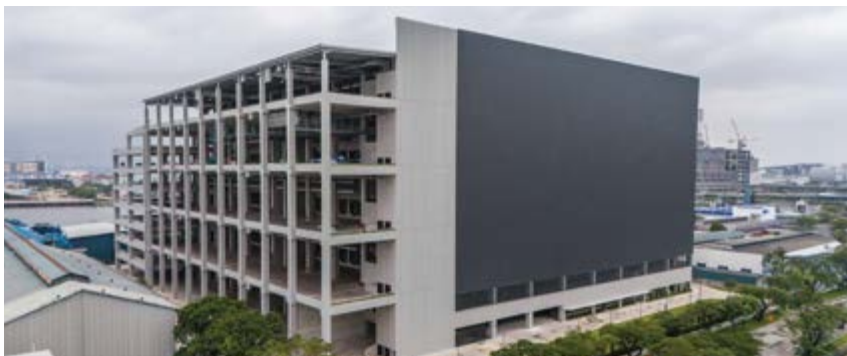
The new warehouse development at 36 Tuas Road
