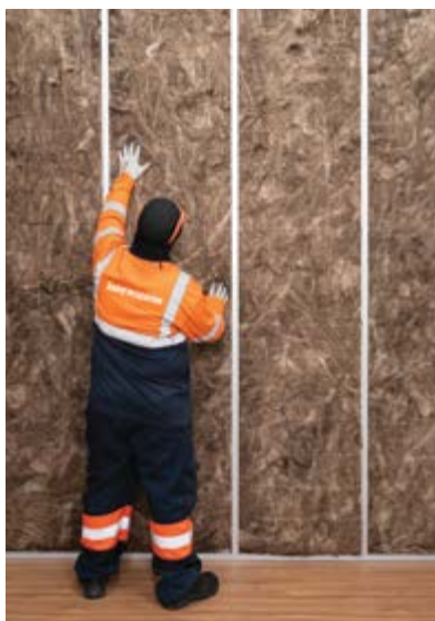
Full height, folded batt internal partition insulation from Knauf Insulation.
