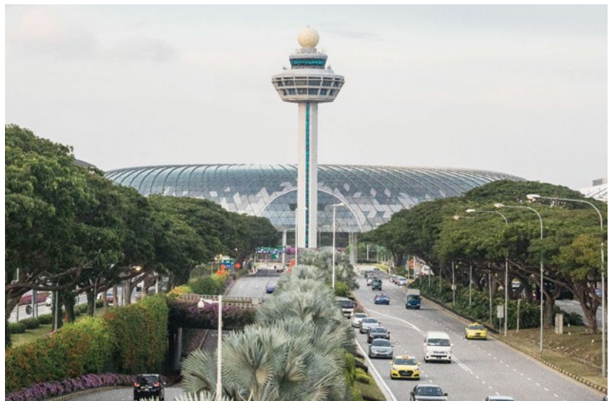
The current Changi Control Tower. Image: Changi Airport Group.
