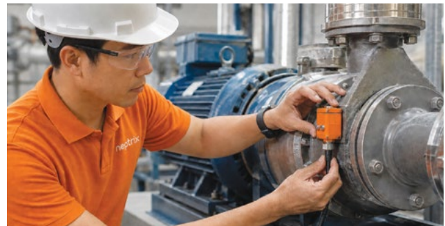
Engineer retrofitting conventional equipment with a smart sensor to extend predictive maintenance.
