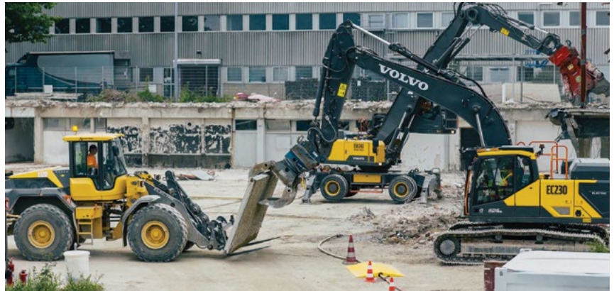
A fleet of all-electric construction machines was successfully deployed to deliver high-performance demolition at the Siemens site.
