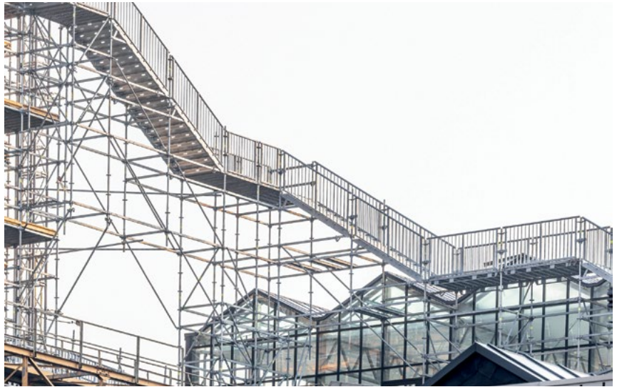
A special feature of the staircase design is the 90° angle at which the stairs wind around the building.
