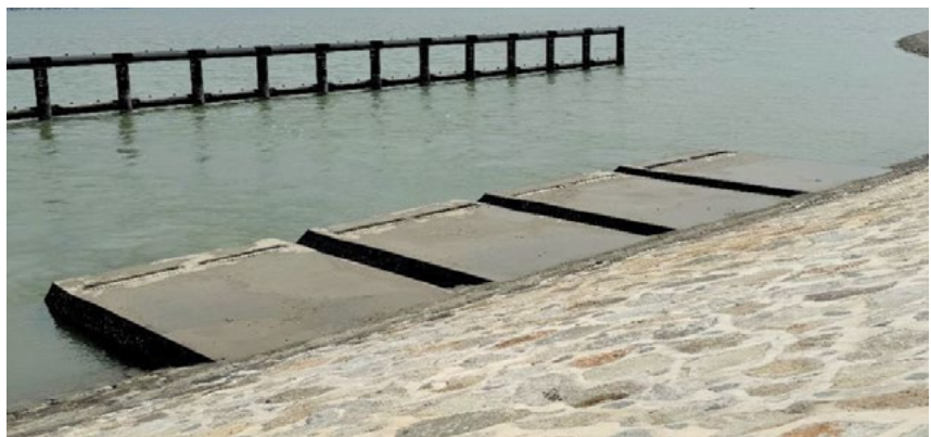
Multiple outlet structures run through the coastal dike and help channel excess water from the polder out into the sea.
