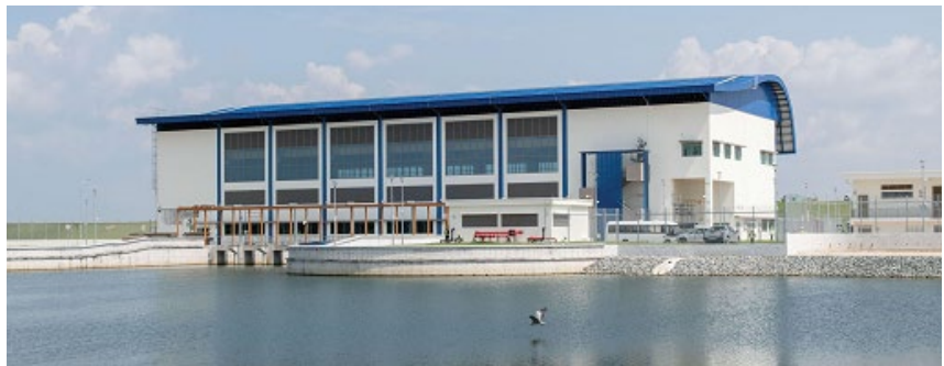
Drainage Pumping Station. Image: PUB, Singapore's National Water Agency.
