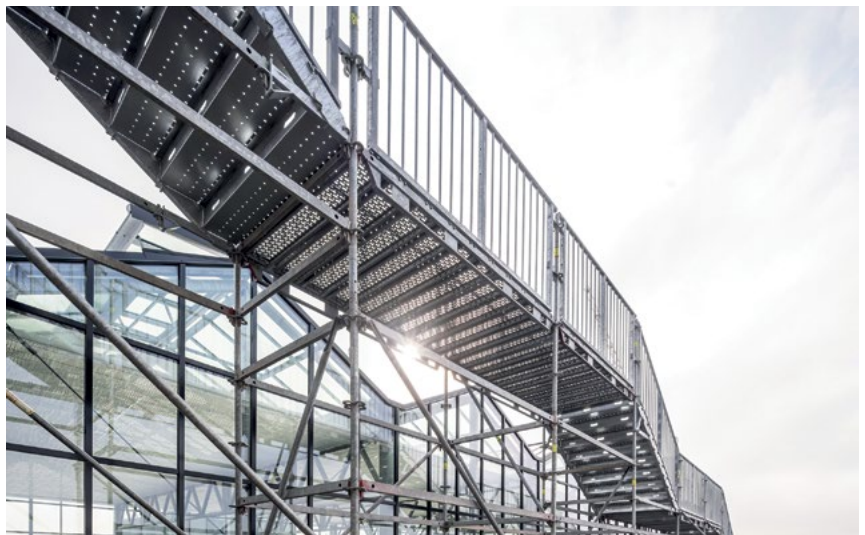
For convenient public access, the PERI UP Public Stair has straight intermediate sections.
