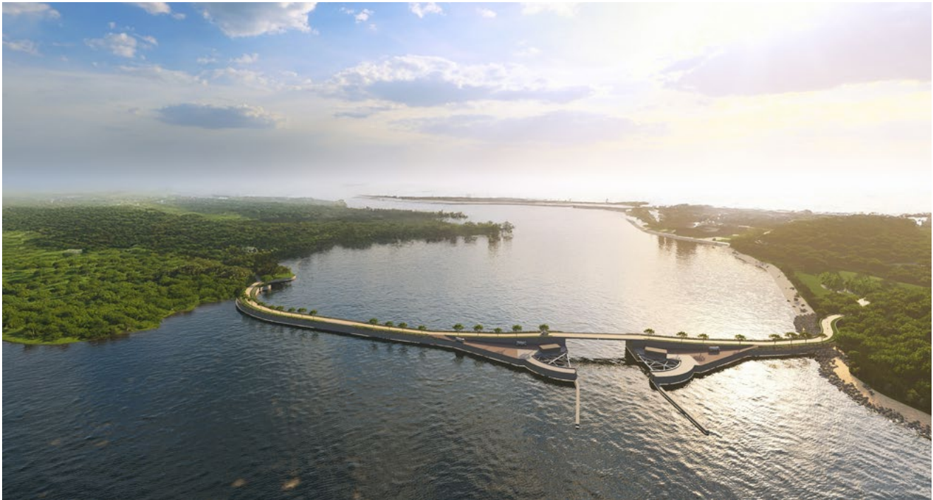
The coastal barrier concept which combines flood protection with enhanced transport connectivity between Sentosa and Pulau Brani. Artist's impression.
