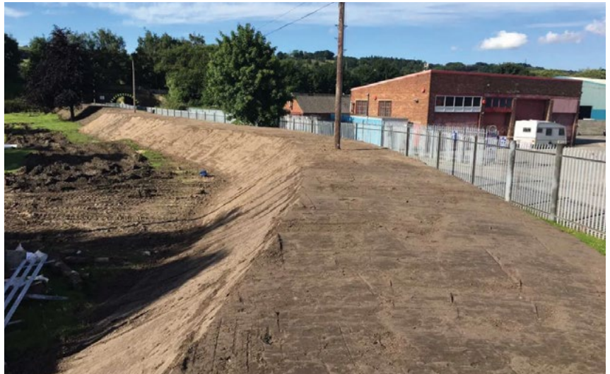
Earth bund in Huddersfield, England. Image: KDSconstruction. ( www.kdsconstruction.co.uk/project/flood-defense-earth-bund/ ).
