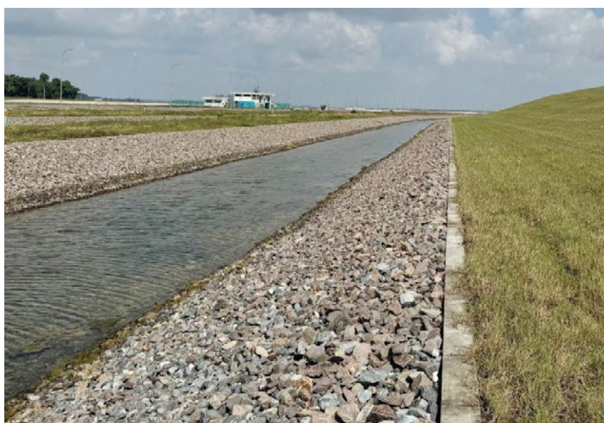
The seepage drain on the landward side of the coastal dike.
