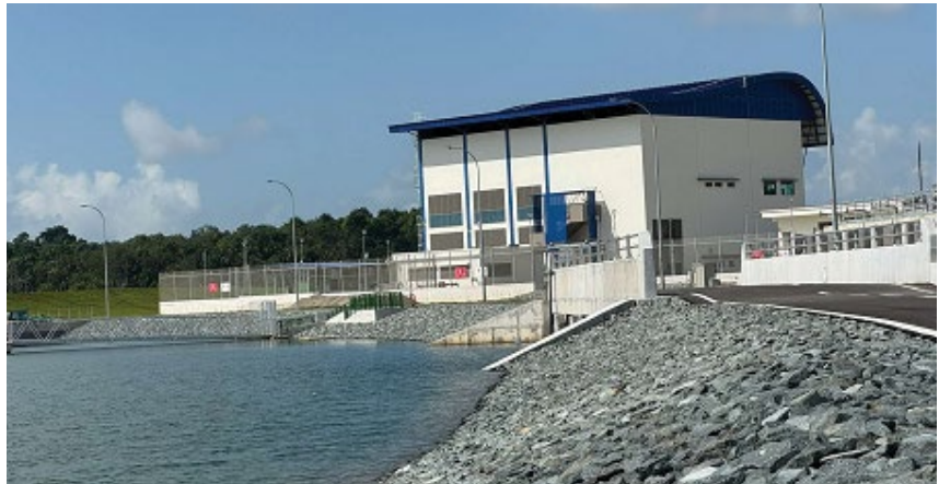
Central Pumping Station.
