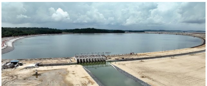
Stormwater collection pond.
