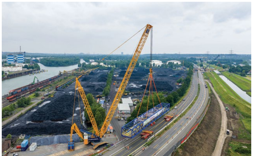
The new bridge segments are moved on SPMTs to the installation area on the closed-off A42.
