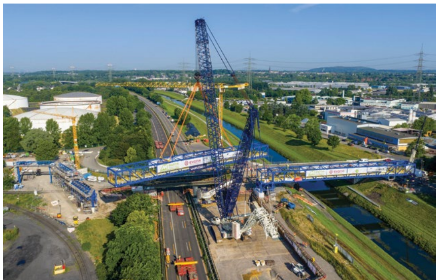
Two steel segments replace four pieces of concrete over the A42 motorway and the River Emscher.
