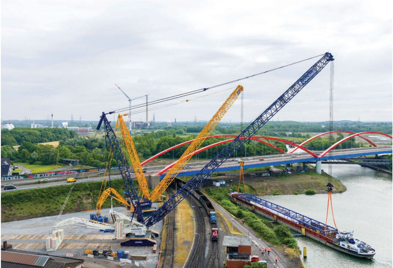
Two Liebherr LR 11000 models unload the first segment of the new pipe bridge from a ship on the Rhine-Herne Canal.
