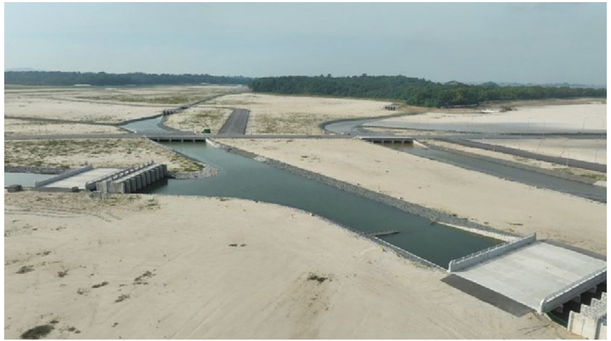
Drainage network on the polder.
