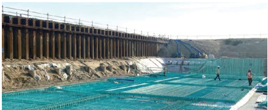
Cofferdams installed to keep construction areas dry.
