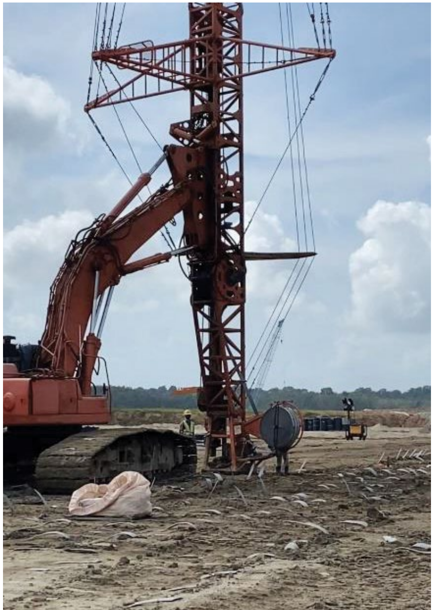
Prefabricated Vertical Drains were inserted to drain water out of the clayey soil.
