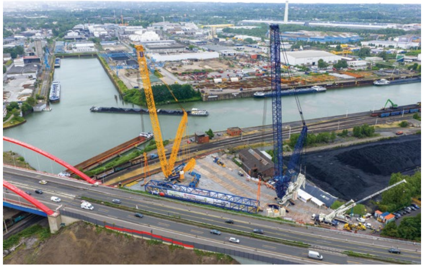
To set down the steel structure, it had to be manoeuvred between both of the crawler cranes. The blue LR 11000 had to be moved several metres under load at the same time.
