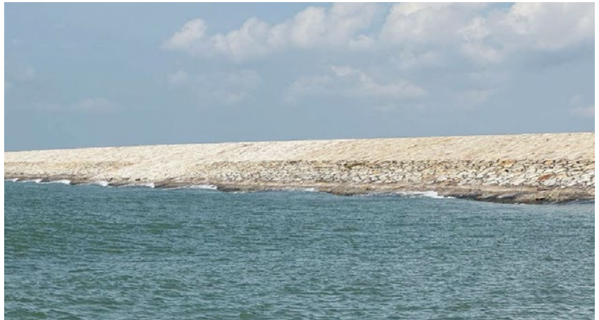
The natural rock layer covering the seaward side of the coastal dike's wall sensitively integrates the polder's coastline with its natural surroundings.
