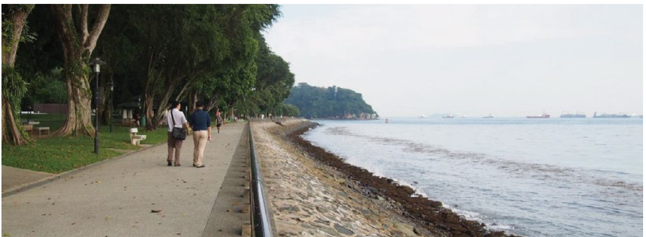
Existing revetment along the coast of Labrador Park.
