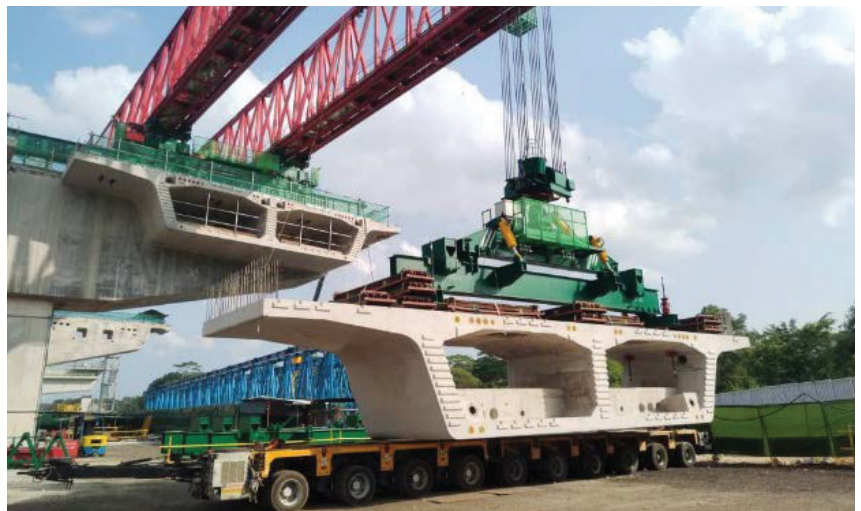
Automated launching gantry for NSC viaduct by China Civil Engineering – China Railway 11 – Wai Fong Consortium.
