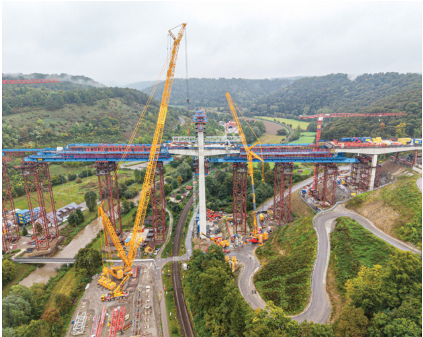
Wiesbauer used two Liebherr cranes to lift reinforcing plates onto the carriageway of the Horb high bridge at a height of 65 m.
