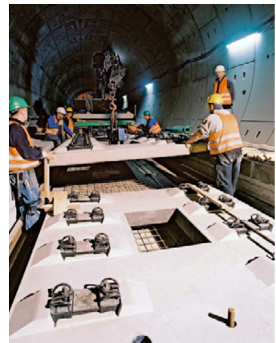
Installation of precast modular slab panels during a tunnel track renewal project. Such methods allow rapid replacement within tight engineering windows. Image: PORR Bau GmbH.
