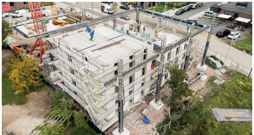
Each DREIHAUS is divided into two segments. While one half is being printed, the ceiling is already being concreted in the other. This allows the multi-family houses to rise quickly. Image: PERI 3D Construction.
