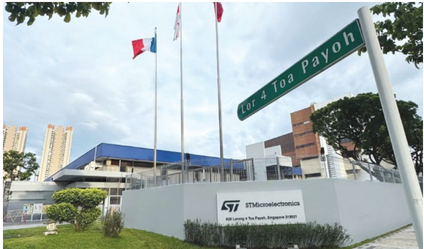
Developed with SP Group, a new chiller cooling system with dual-temperature capability, at STMicroelectronics Toa Payoh, will optimise energy usage and reduce about 2,140 tons of carbon emissions annually.
