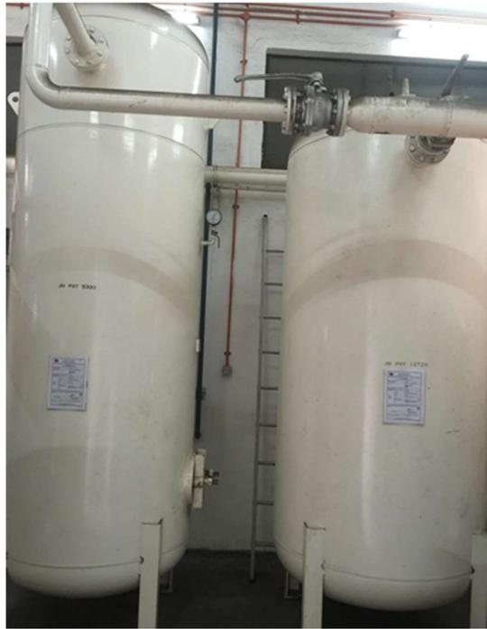
Figure 7.6 Air receiver tanks
