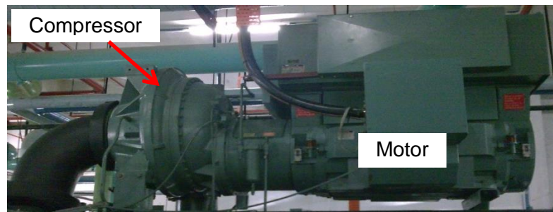
Figure 1.17 Photograph of an open-type compressor system
