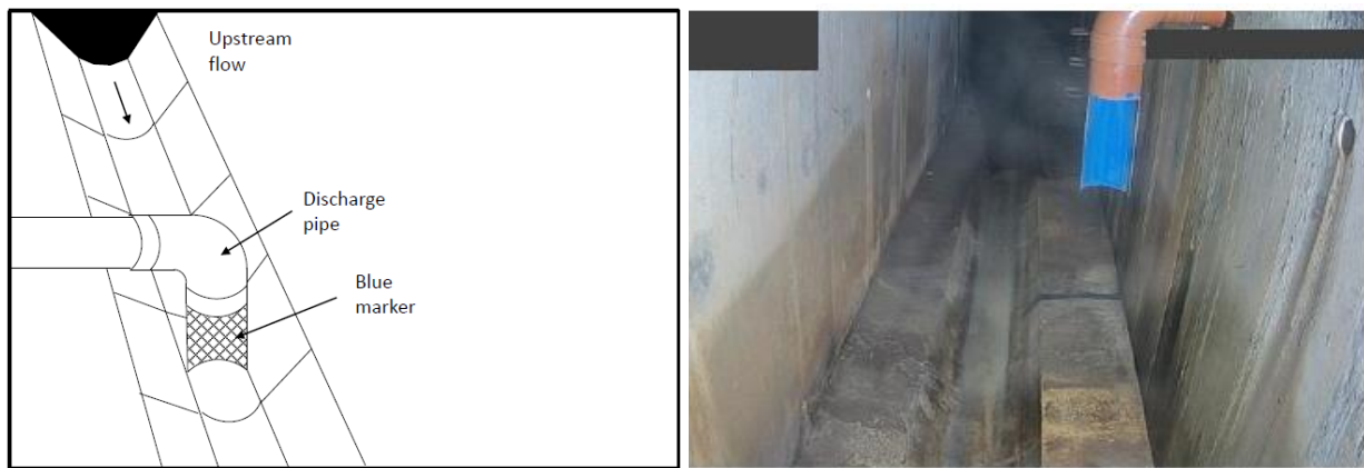
Figure 2. Example of Blue-Marker painted on cut-opened discharged pipe.
