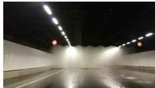
Overhead water sprinkler system in tunnels
