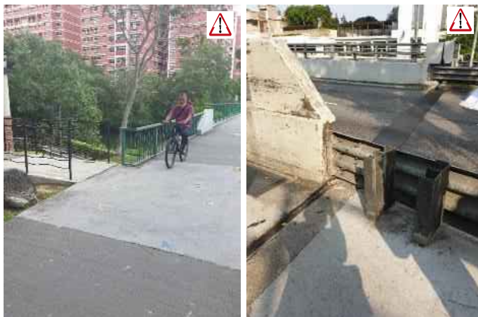
Figure 4.41: Examples of poor restraint structures
