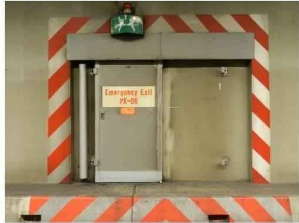
Pedestrian cross passage door (every 100m, next to fast lane)
