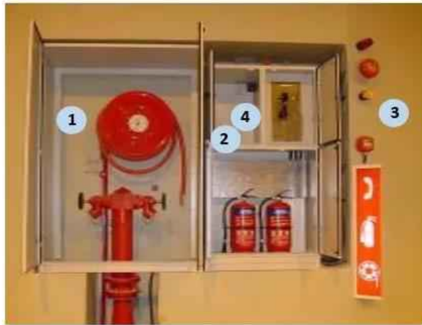
Figure 4.75: Fire Service cabinet equipment
