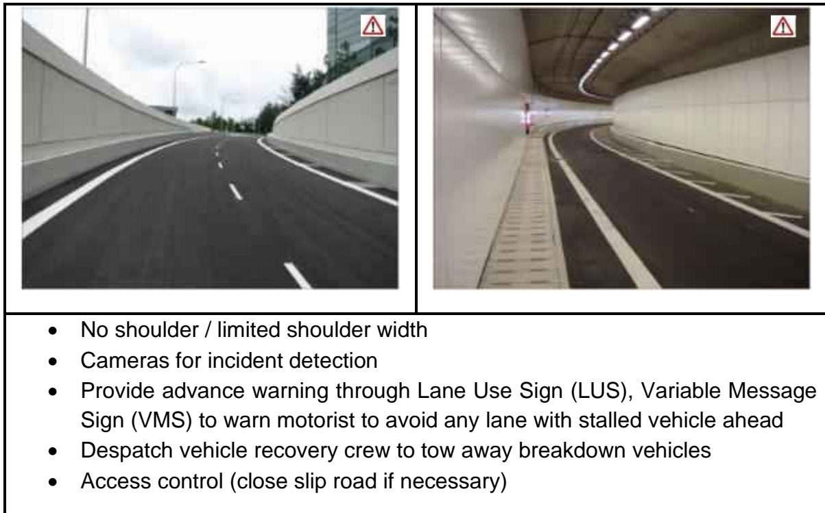
Figure 4.11: Substandard shoulder width
