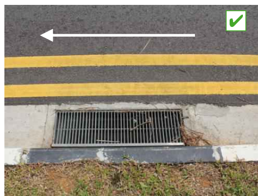
Figure 4.15: Provision of drainage inlets with gratings that are perpendicular to the direction of travel and smaller gaps in-between the gratings
