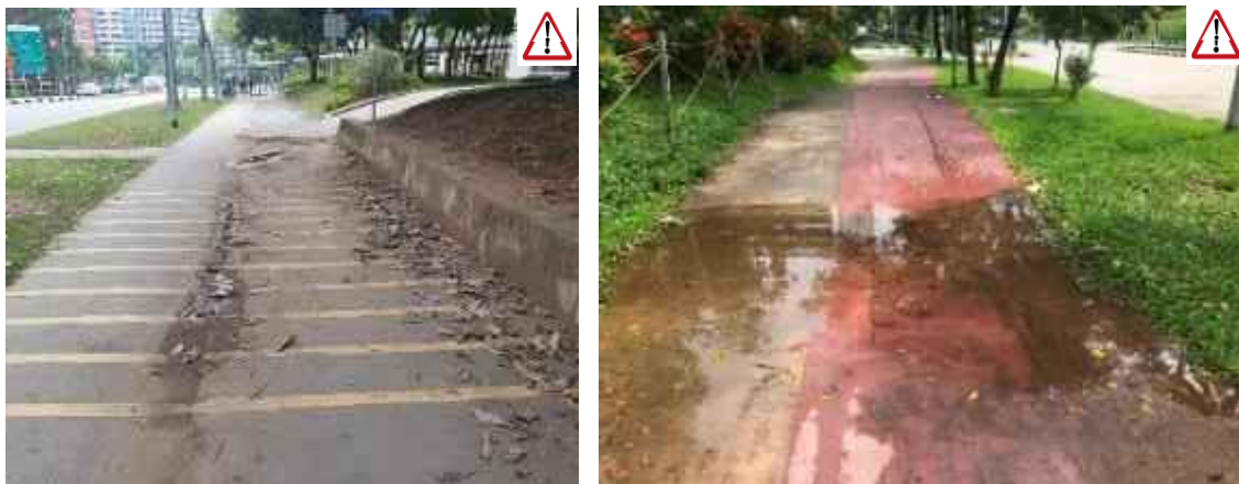
Figure 4.40: Poor drainage causing water ponding at path
