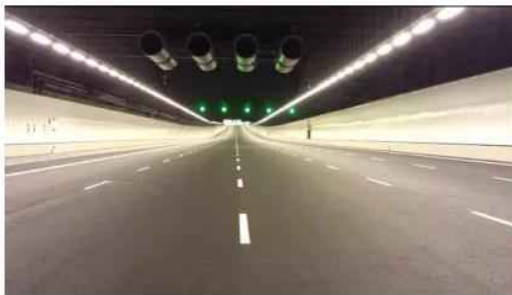
Ventilation system in the tunnel
