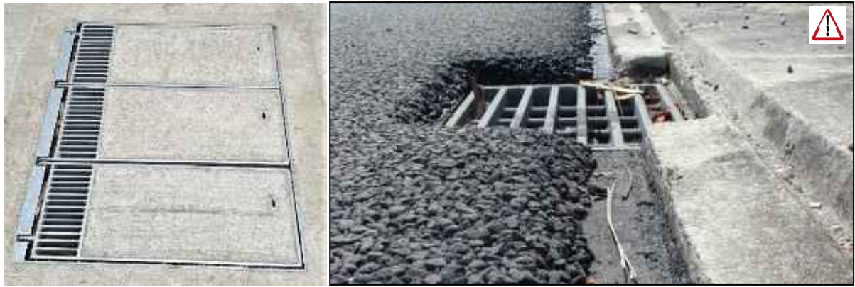
Figure 4.39: Good and poor example of drain grating
