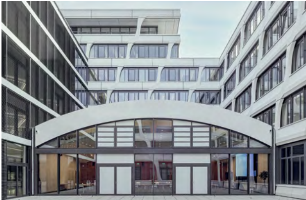
For the dome ceiling, PERI developed a formwork solution made with 82 factory pre-assembled, 3D-designed architectural concrete timber formers that were delivered pre-assembled to the construction site.
