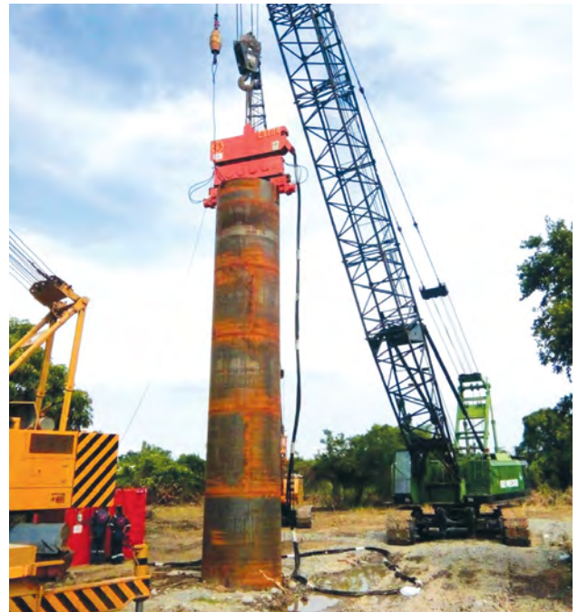
A 5-ton series normal frequency crane suspended hydraulic vibratory hammer.
