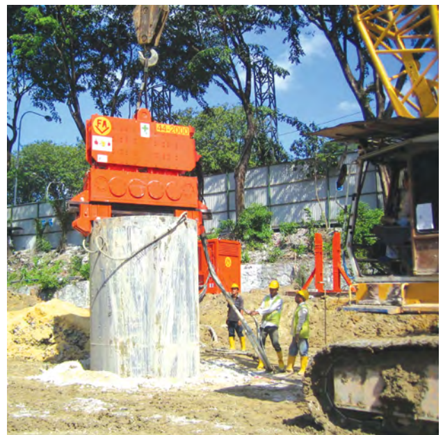
An 8-ton series high frequency crane-suspended hydraulic vibratory hammer at work.
