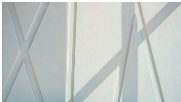
The feature wall consists of several prefabricated concrete elements. These were subsequently mounted to the in-situ concrete wall.
