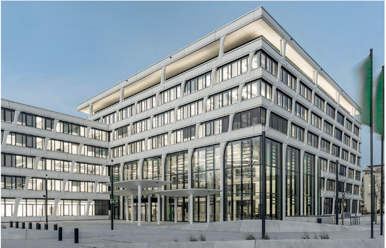
An exterior view of the building. The 11.75 m high facade supports were realised with PERI timber girder formwork.
