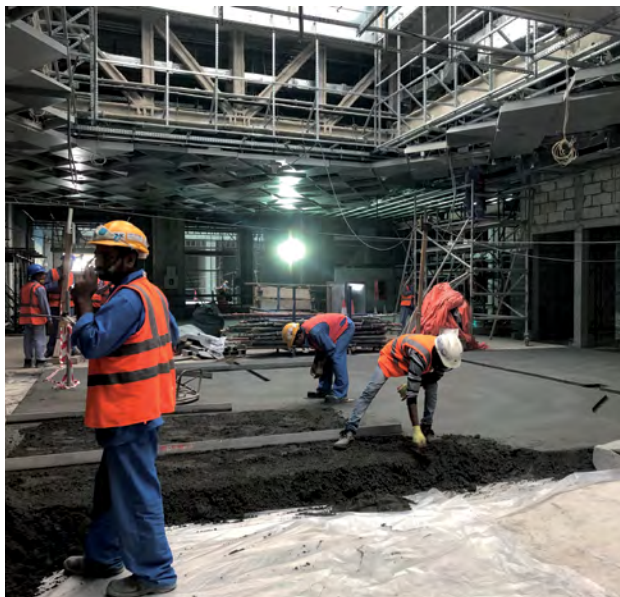
TOPCEM hydraulic binder was used to create the rapid-drying screeds in the stations.
