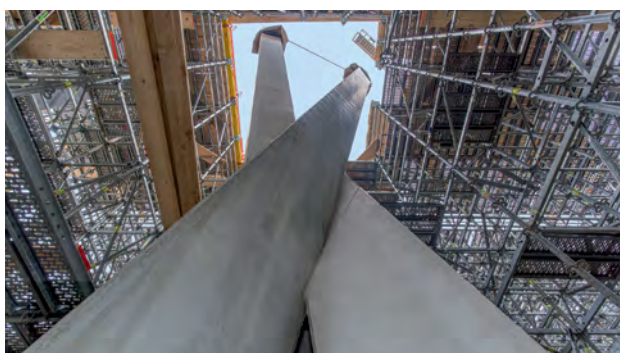
The formwork for the tree supports fitted into the already erected PERI UP Shoring without any problems. Image: PERI AG.
