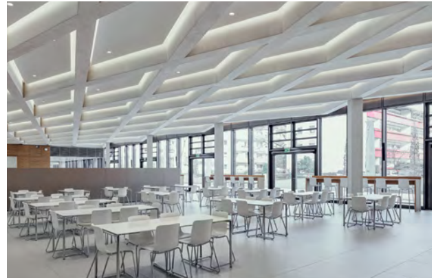
For the casino slab, PERI special formwork developed especially for the project was used, which was later fitted with a total of 64 different, diamond-shaped box outs, pre-assembled in the factory.
