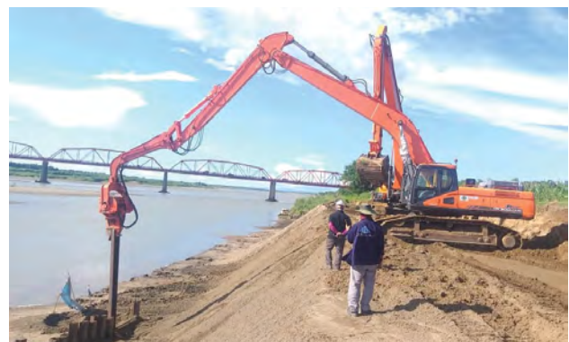
An excavator mounted vibratory hammer, with extended boom, driving a sheetpile as part of a flood control project in Philippines.
