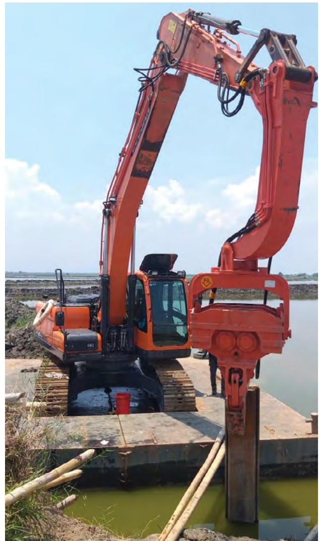
An excavator mounted vibratory hammer driving a sheet pile into a targeted area.
