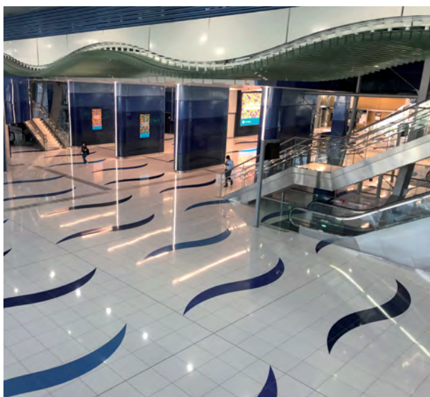
In the stations, the engineered stone flooring was installed with GRANIRAPID before grouting joints with KERACOLOR FF + FUGOLASTIC.
