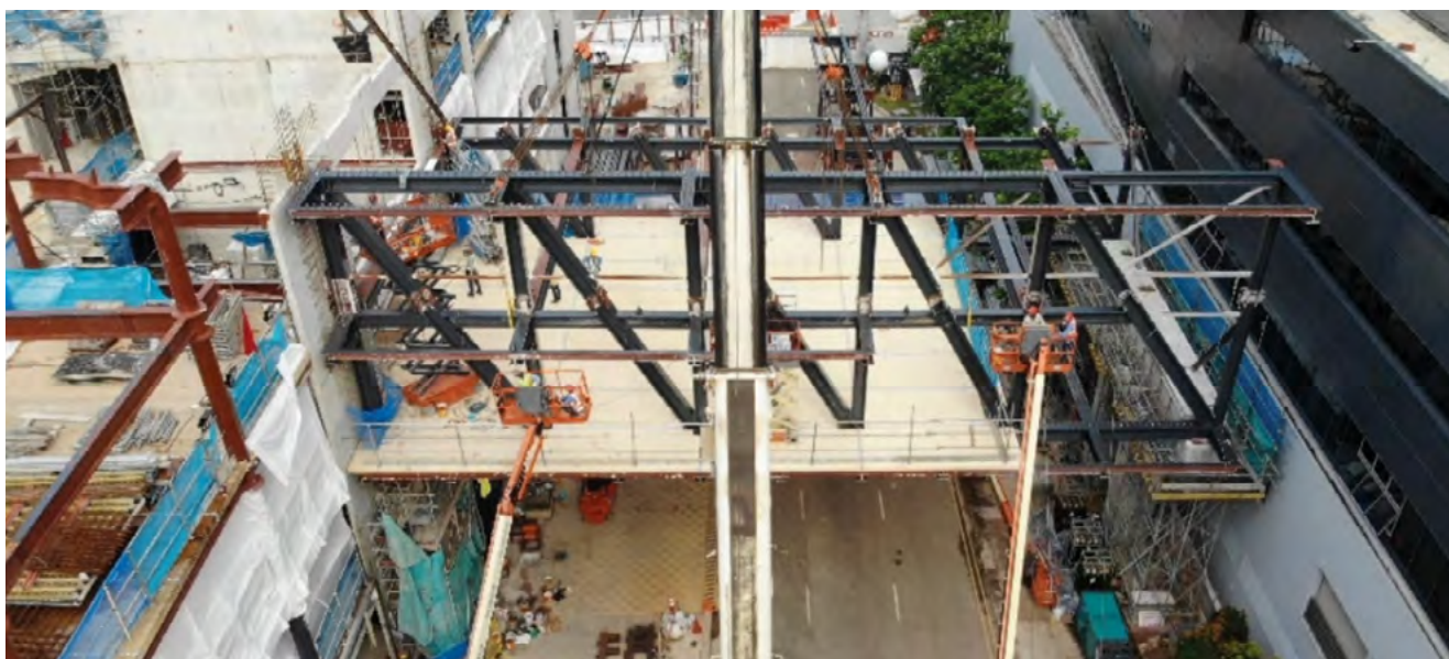
Welding of truss segments and installation of CLT panels.
