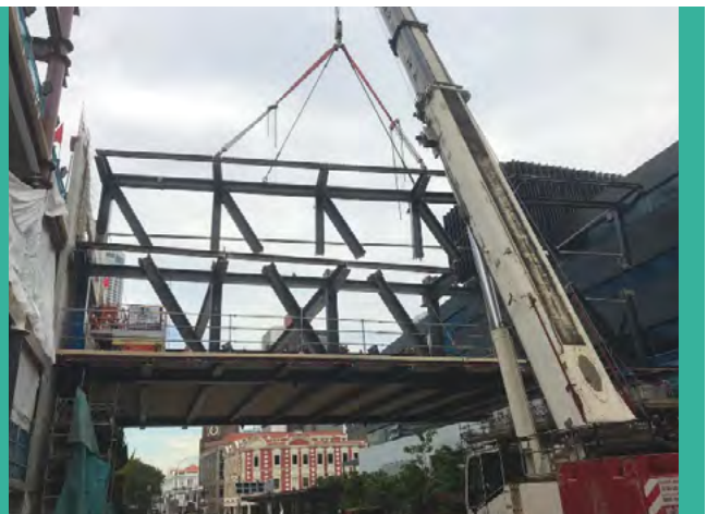
Installation of lower truss segments.
