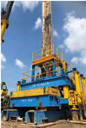
Figure 3: Installation of Hat+H piles using the jack-in press-in method.
