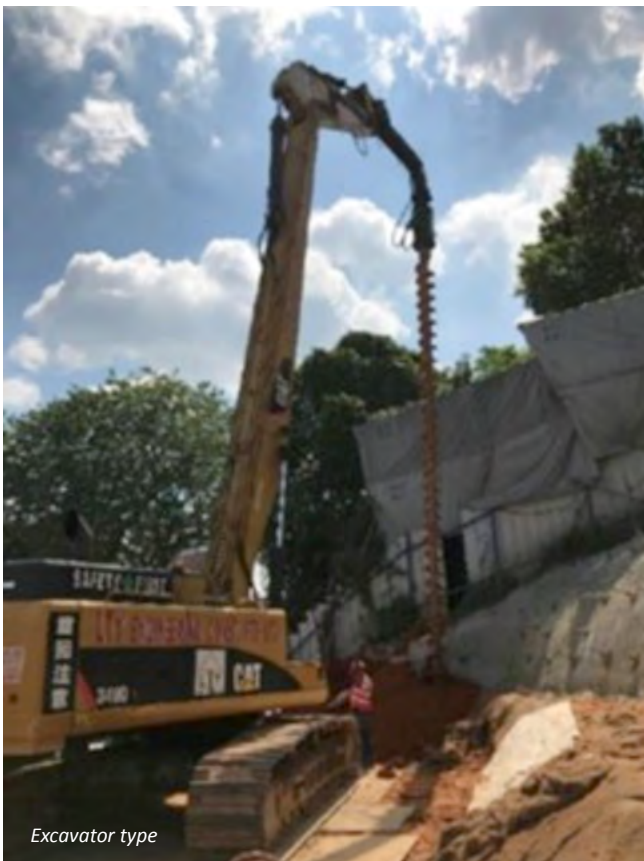
Picture 4: Pre-augering in hard soil layers.
