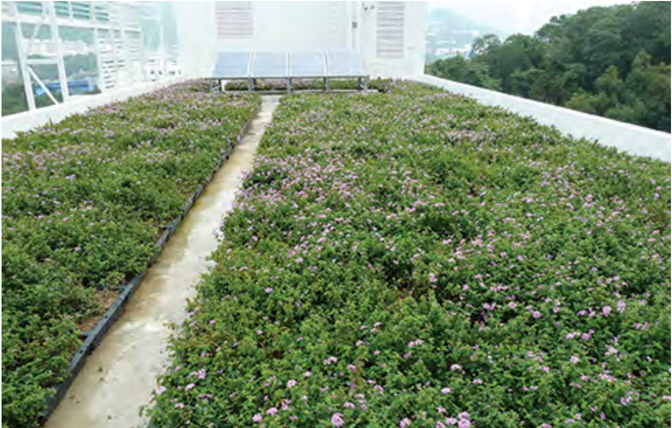
The PEG Roof Tray System helps to green the rooftops of buildings, thereby addressing the environmental concerns of many cities with limited green spaces.
