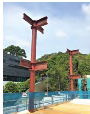
Prefabricated structural steel beam-column frames erected on site.
