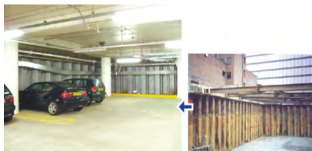
Picture 2: Application of Hat solutions as an underground permanent wall. Image: Giken ASIA.
