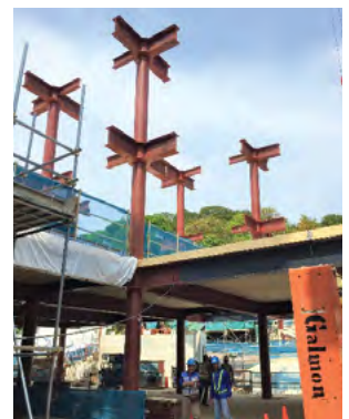
Prefabricated structural steel beam-column frames erected on site.
