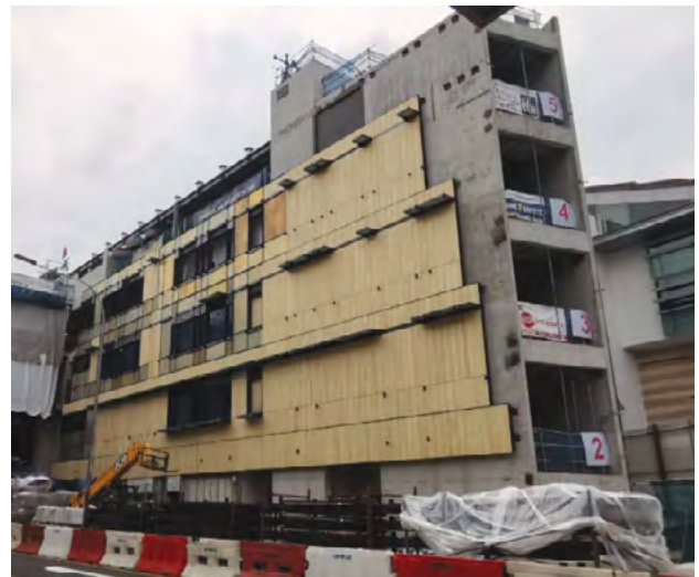
Installation of the DfMA façade.
