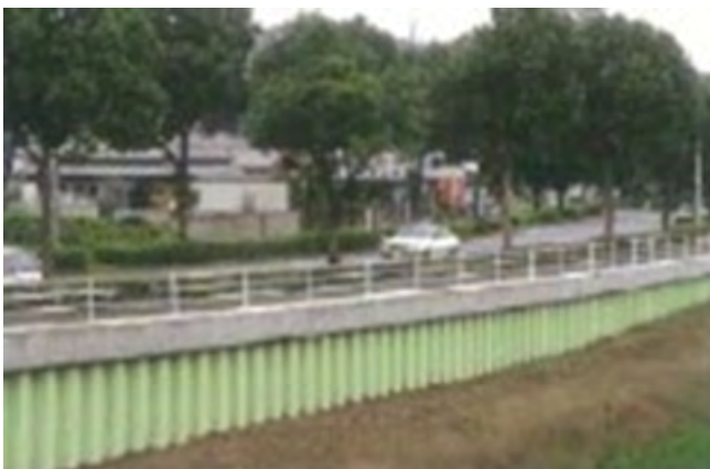
Picture 3: Actual application of Hat solutions as permanent retaining wall.
