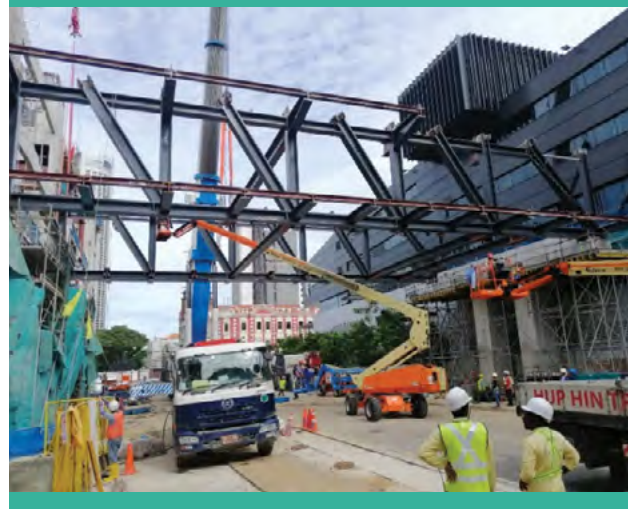
Installation of lower truss segments.
