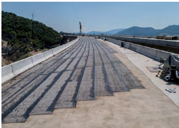
Waterproofing the road surfaces with Polyglass solutions.
