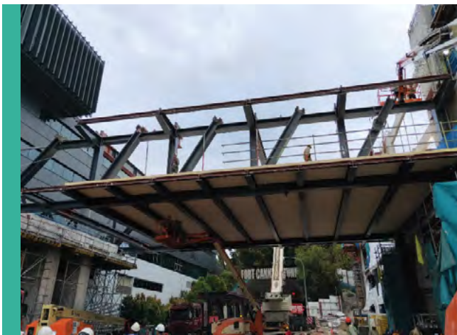
Installation of CLT panels and upper truss segment.
