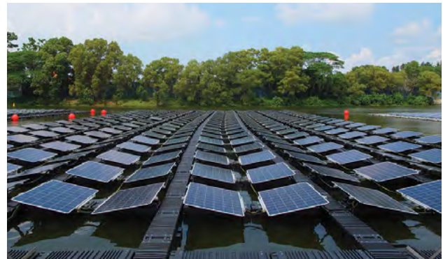
The FSS holds solar panels on water bodies to harvest solar energy.
