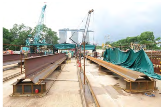
Picture 1: The Hat+H combined pile has been installed in an MRT station portion, as a temporary wall, and then it was extracted after around three years.
