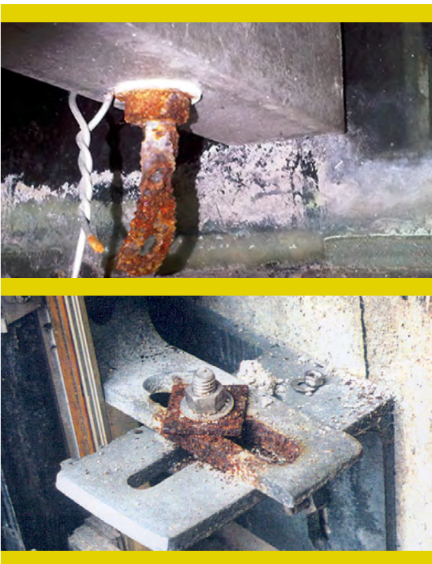
Corroded fixing (above) and steel bracket (below).
