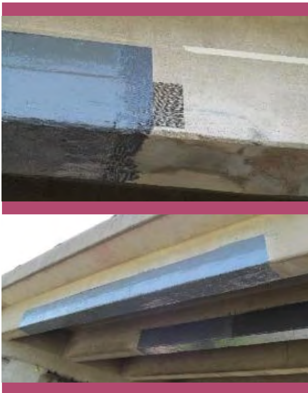
Figure 3: Impacted RC girder retrofit - finger joint of CRP 070 left void of epoxy (image on top) and completed repairs following UV protective coating (image below).
