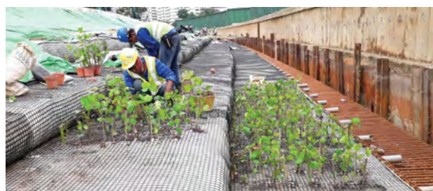
Figure 5: Geogrid-geotextile combination facing that has been completed for the project, with plants starting to grow on it.
