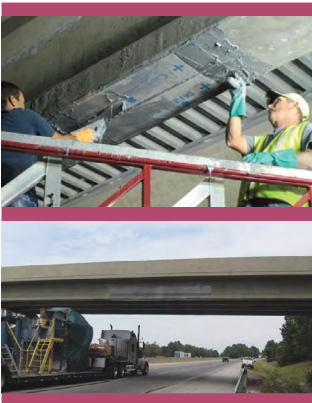
Figure 5: Impacted PC girder retrofit - CRP 195 application (image on top) and completed retrofit (image below).
