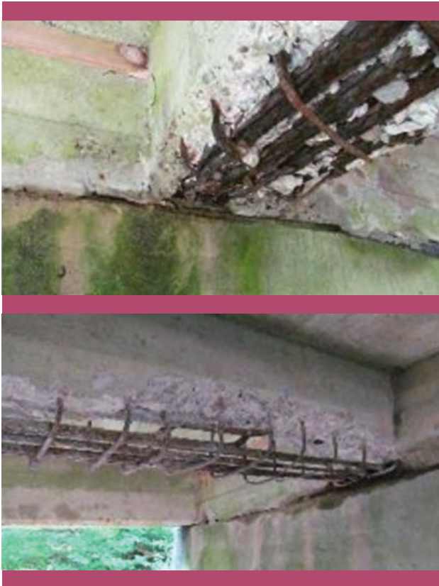
Figure 6: Deteriorated RC girders - corroded rebar (image on top) and after removal of deteriorated concrete (image below).
