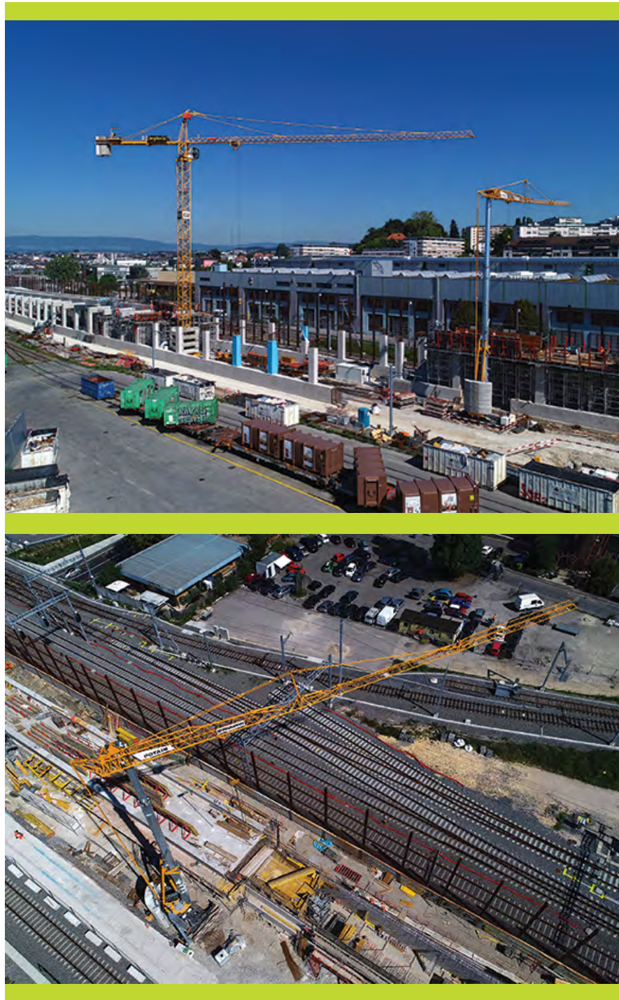
The Potain Hup C 40-30 cranes are working round-the-clock for the construction of the rail flyover.
