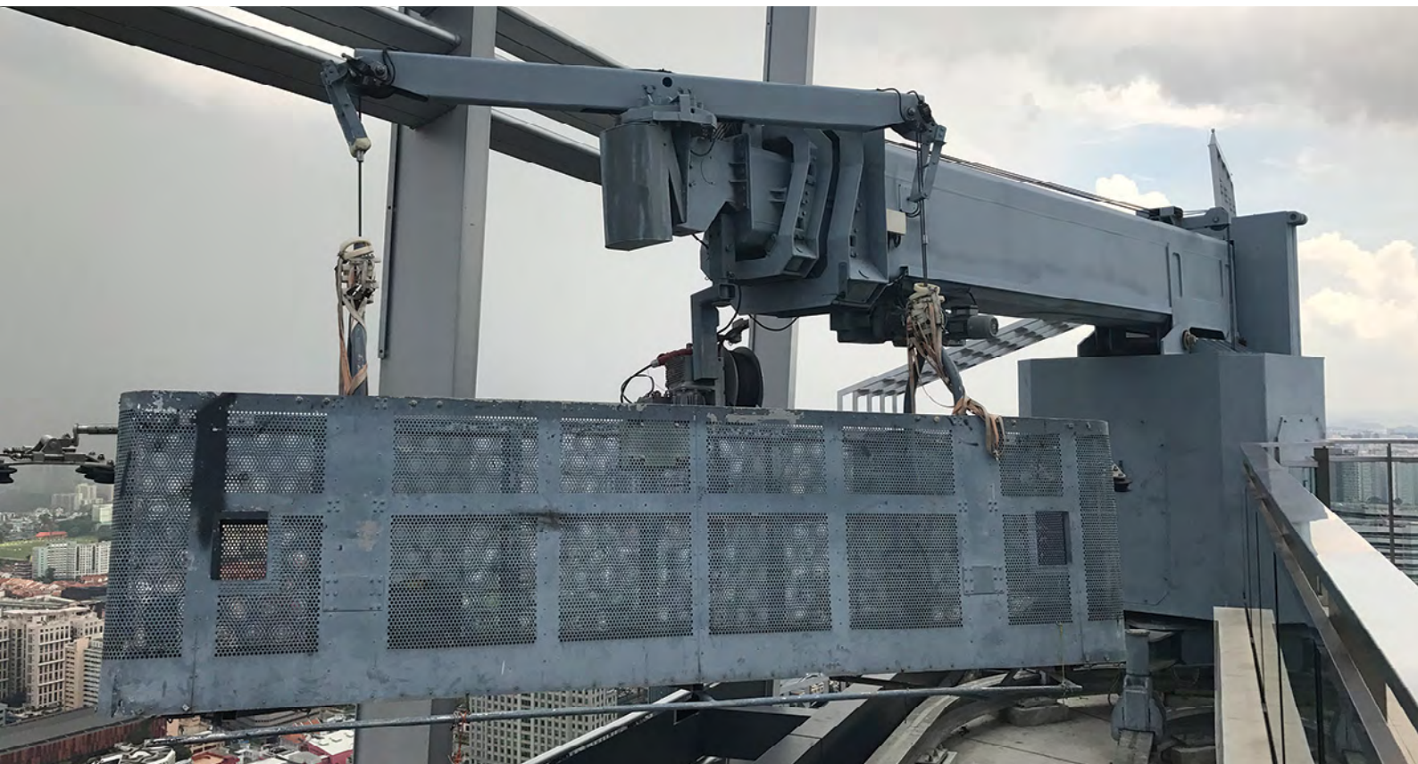
Safe access for inspections using the Building Maintenance Unit (BMU).
