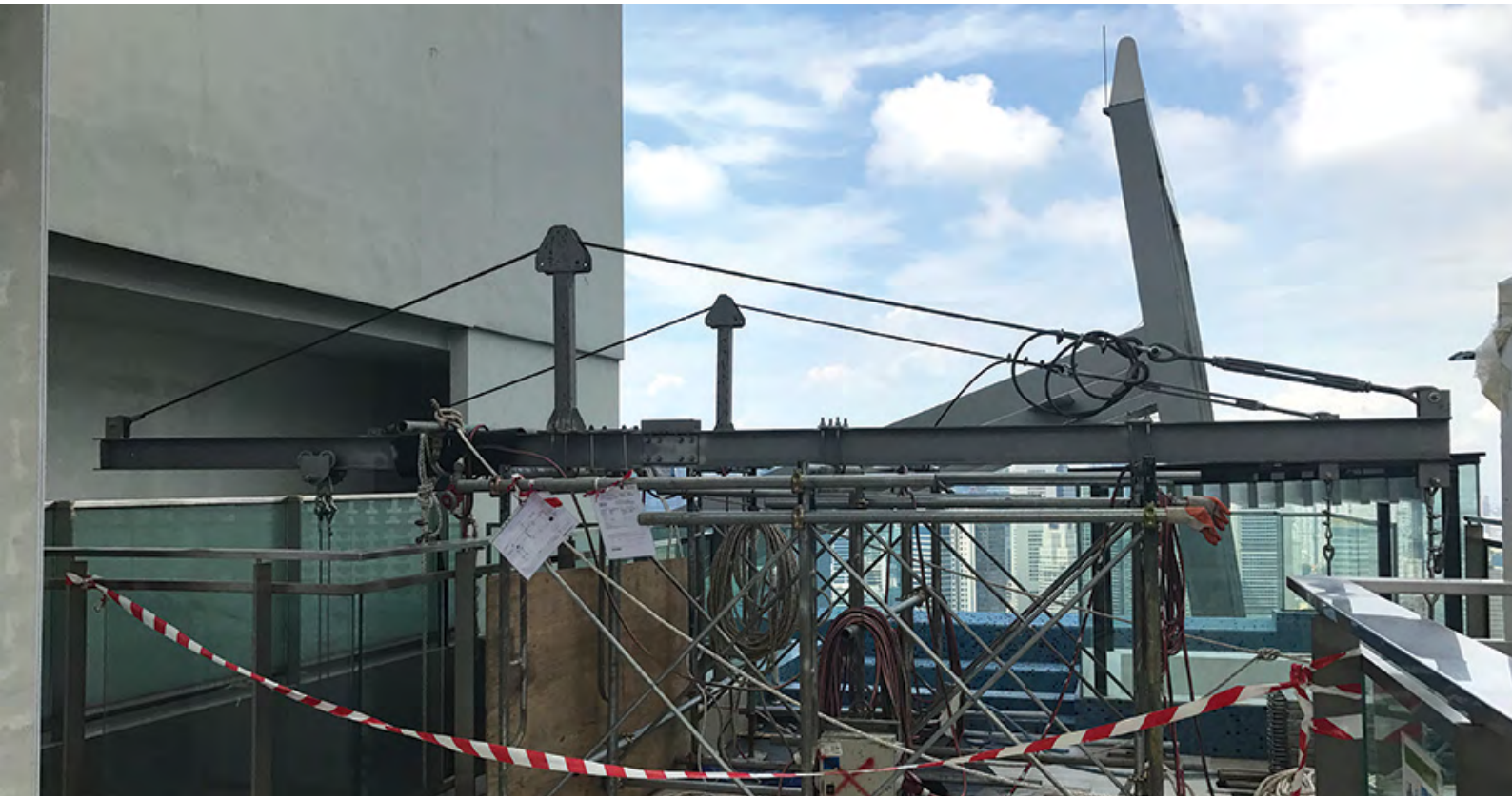
Temporary counter-weight system for façade access.
