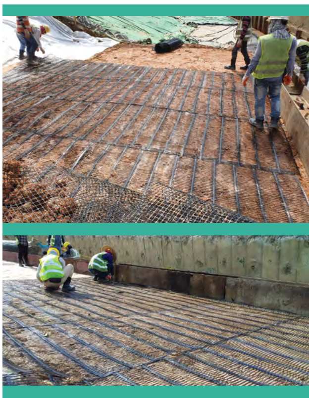
Figure 4: The laying of geogrids by workers is a relatively easy process.
