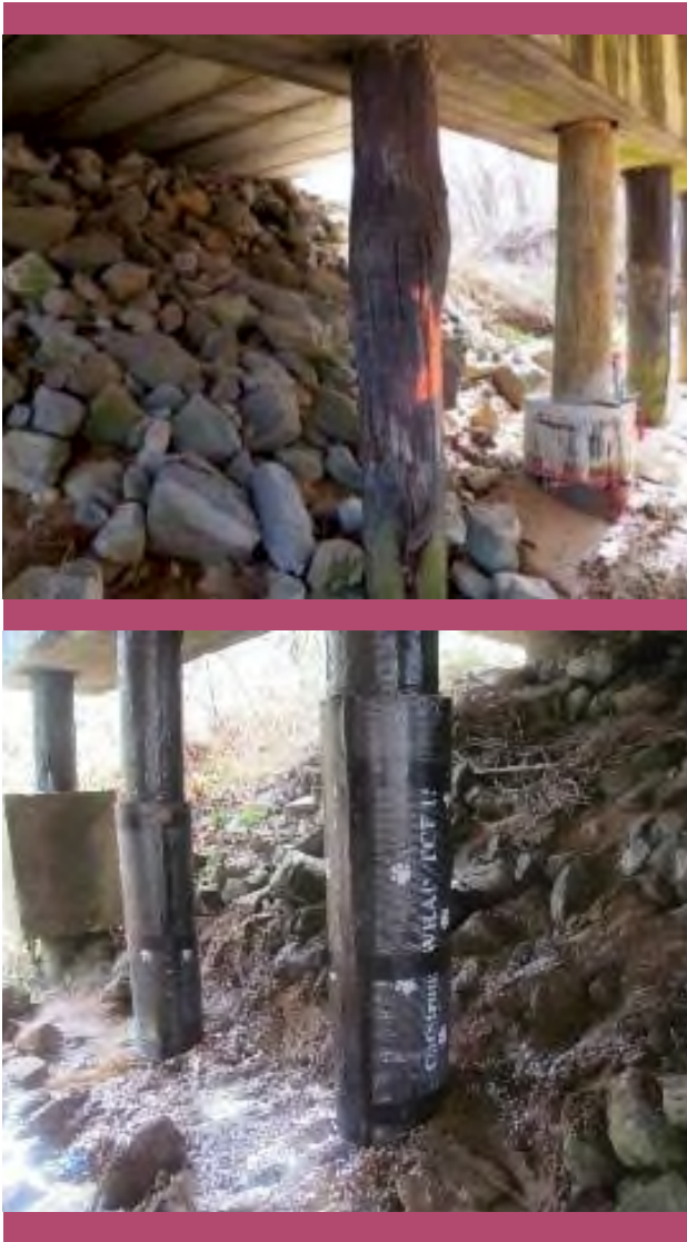
Figure 10: Strengthening deteriorated timber piles - deteriorated pile (image on top) and strengthened PC Box beam ends following CatStrong TCF 012 application (image below).
