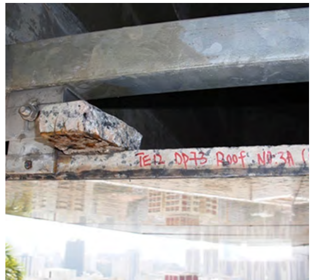
Detached soffit panel.
