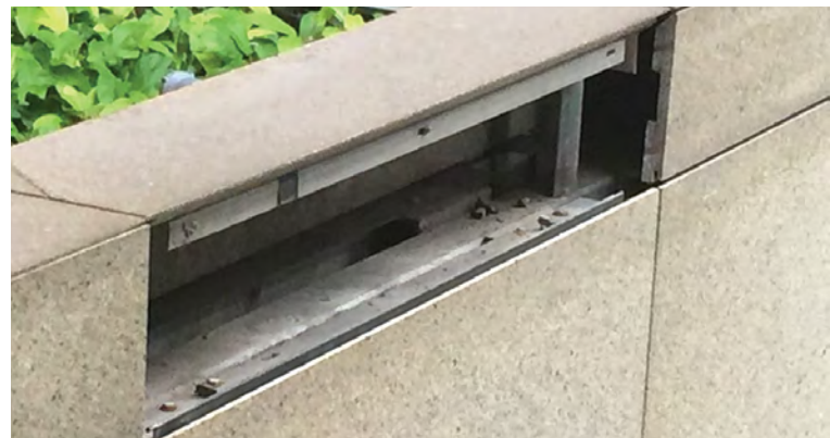
Void created by fallen stone facade panel.
