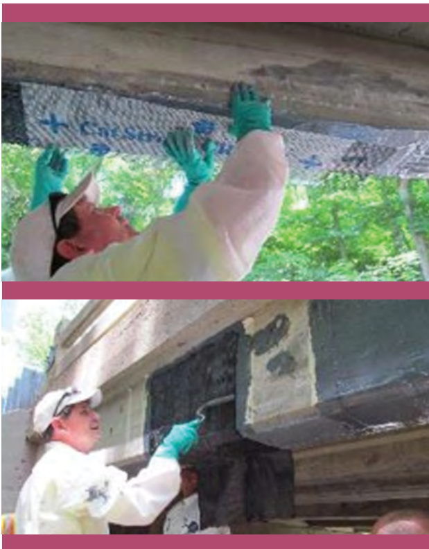
Figure 7: Deteriorated RC girder retrofit -CRP application on bottom surface (image on top) and TCF 012 application over finger joints (image below).
