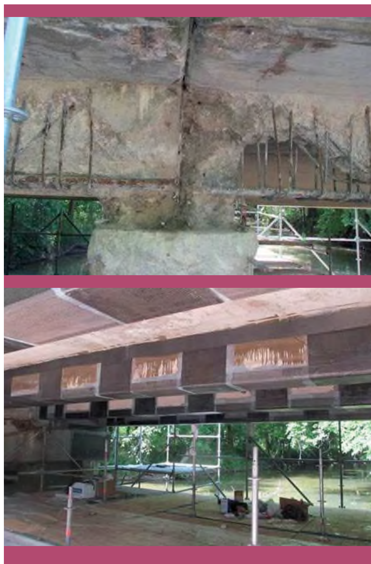
Figure 8: Increasing load-rating of RC bridge - deteriorated pier cap and RC girders (image on top) and RC girders following CatStrong UCF and TCF application (image below).
