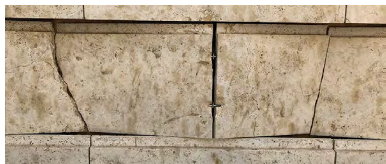
Damaged stone cladding.
