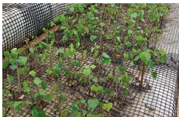
Figure 6: A close-up of the plants growing out from the geogrid-geotextile combination facing.
