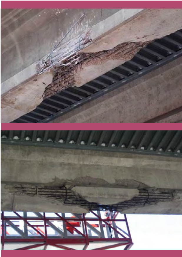
Figure 4: Impact-damaged prestressed concrete (PC) girders.
