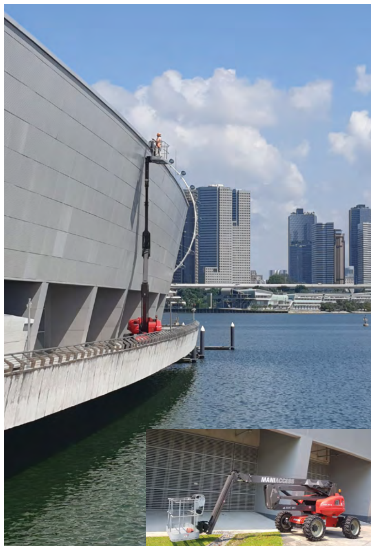
One important application of Manitou machines, in the context of Singapore, is in façade inspection and maintenance, especially in light of the proposed changes to the Building Control Act, that will make façade inspections mandatory for older buildings. Main Image: Fanch-Ronan, Manitou Asia Pte Ltd. Inset Image: Vincent Koay, Manitou Asia Pte Ltd.
