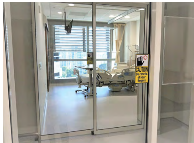
Negative pressure room with double door at NCID. Image: NCID.
